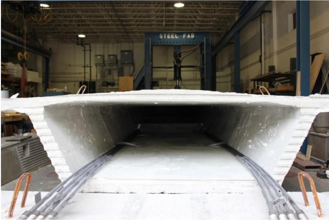
Figure A9. Post-Tensioning Cables through the Segments
