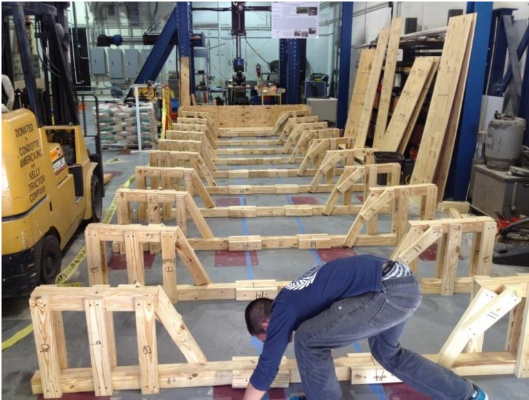
Figure A1. Formwork Framing
