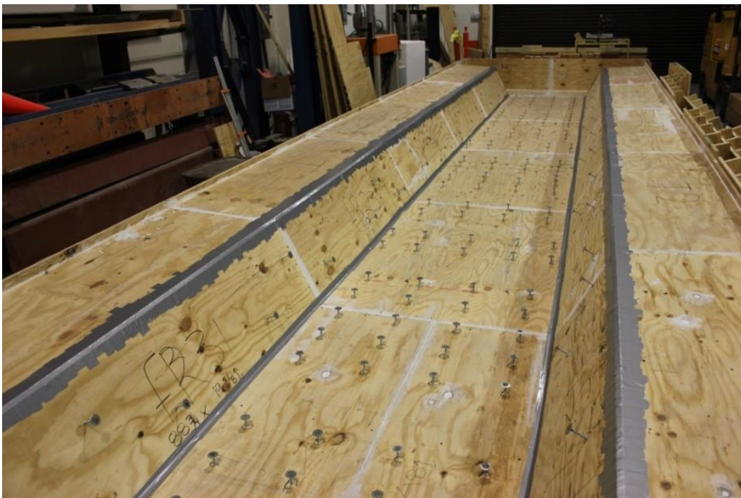
Figure A2. Formwork Base
