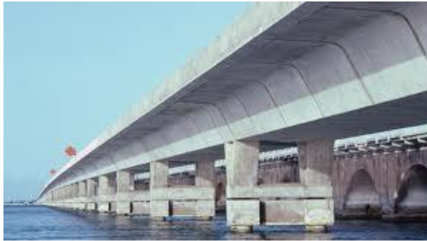
Figure 2.4 Long Key Segmental Bridge in the Florida Keys
