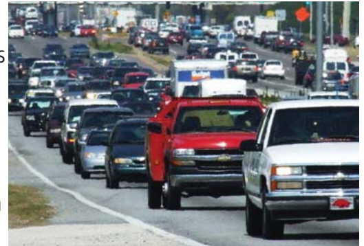
TSM&O can provide management tools that promote greater efficiency of existing roadways.
