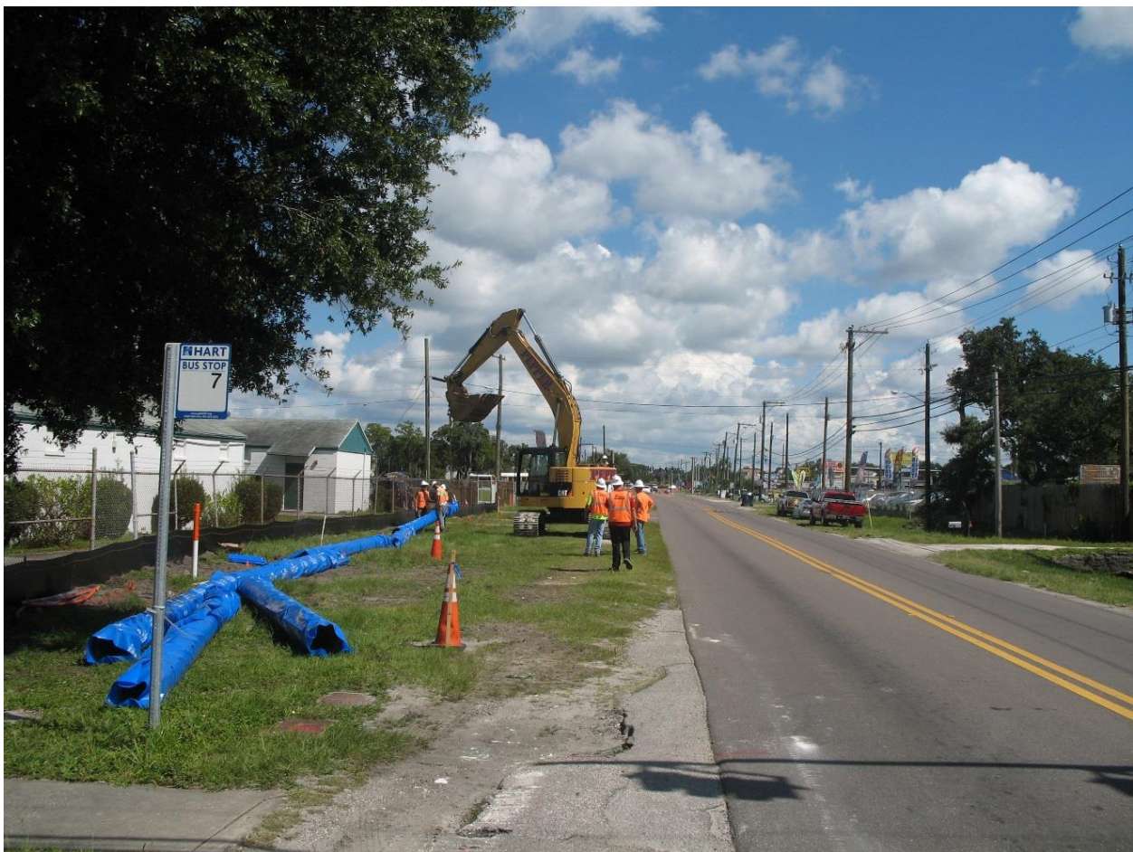
Figure 7-6: Tampa Site Visit
