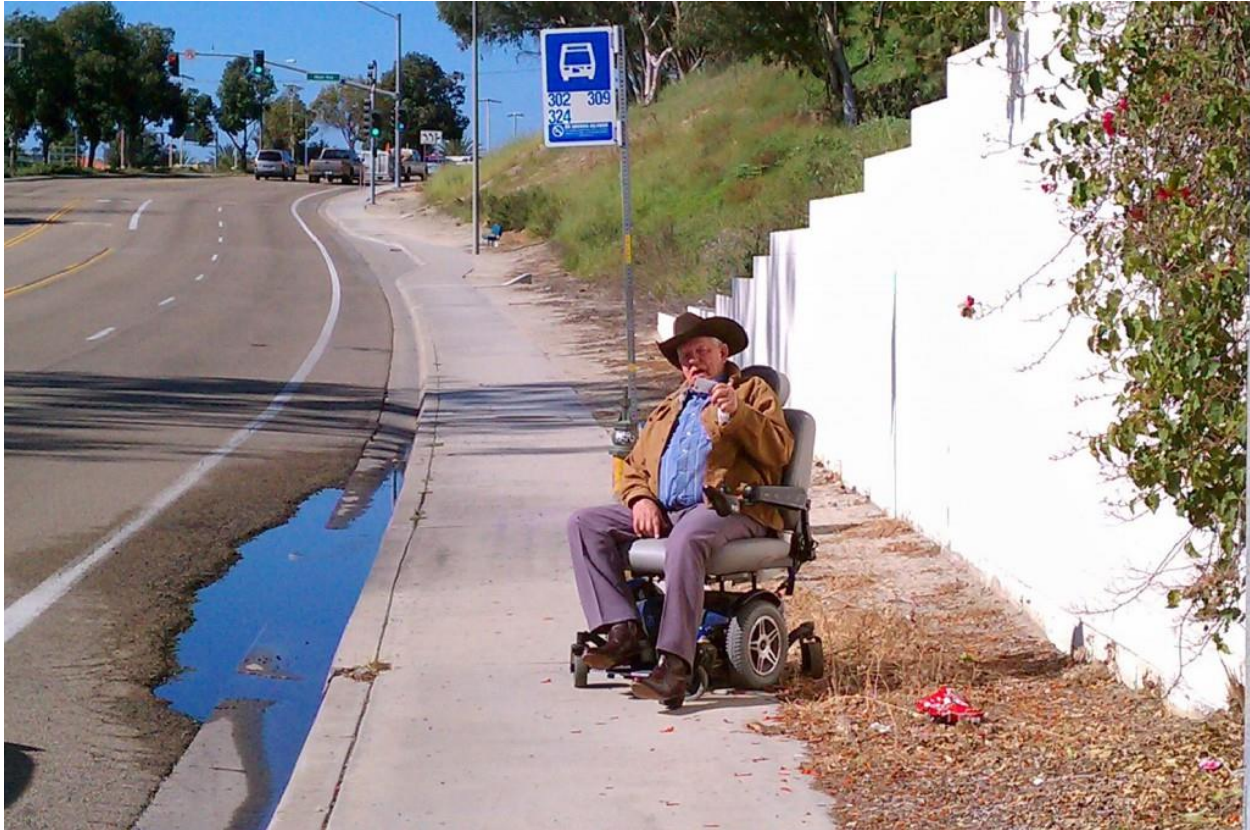
Figure 5-21: Poor Drainage Location at a Bus Stop
