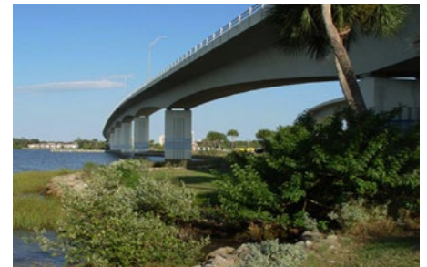
The Seabreeze Bridge in Daytona Beach, Florida, is one of many that use post-tensioned concrete components.
