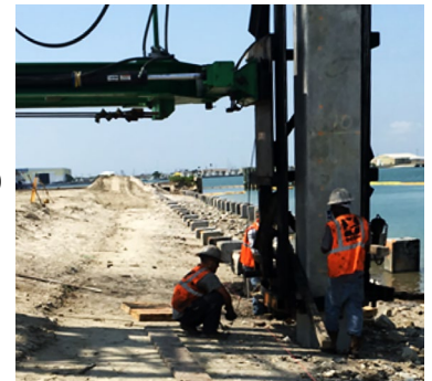
Workers inspect a driven concrete pile.
