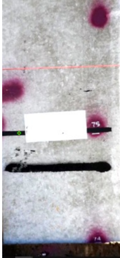
Figure D-6 Dunns Creek Concrete Test Pile Photo at 75-Foot Location from 9/19/2018 Video Frame Recorded At 60-Hz
