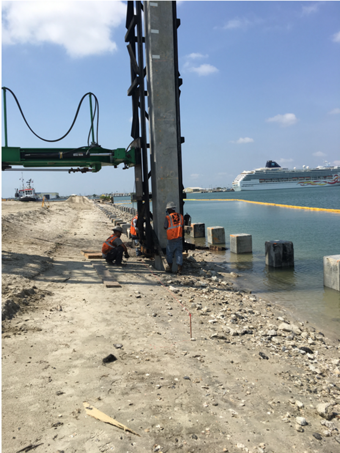
Figure 3-4 North Cargo Berth 8 Pile Driving and Preliminary PDM Testing
