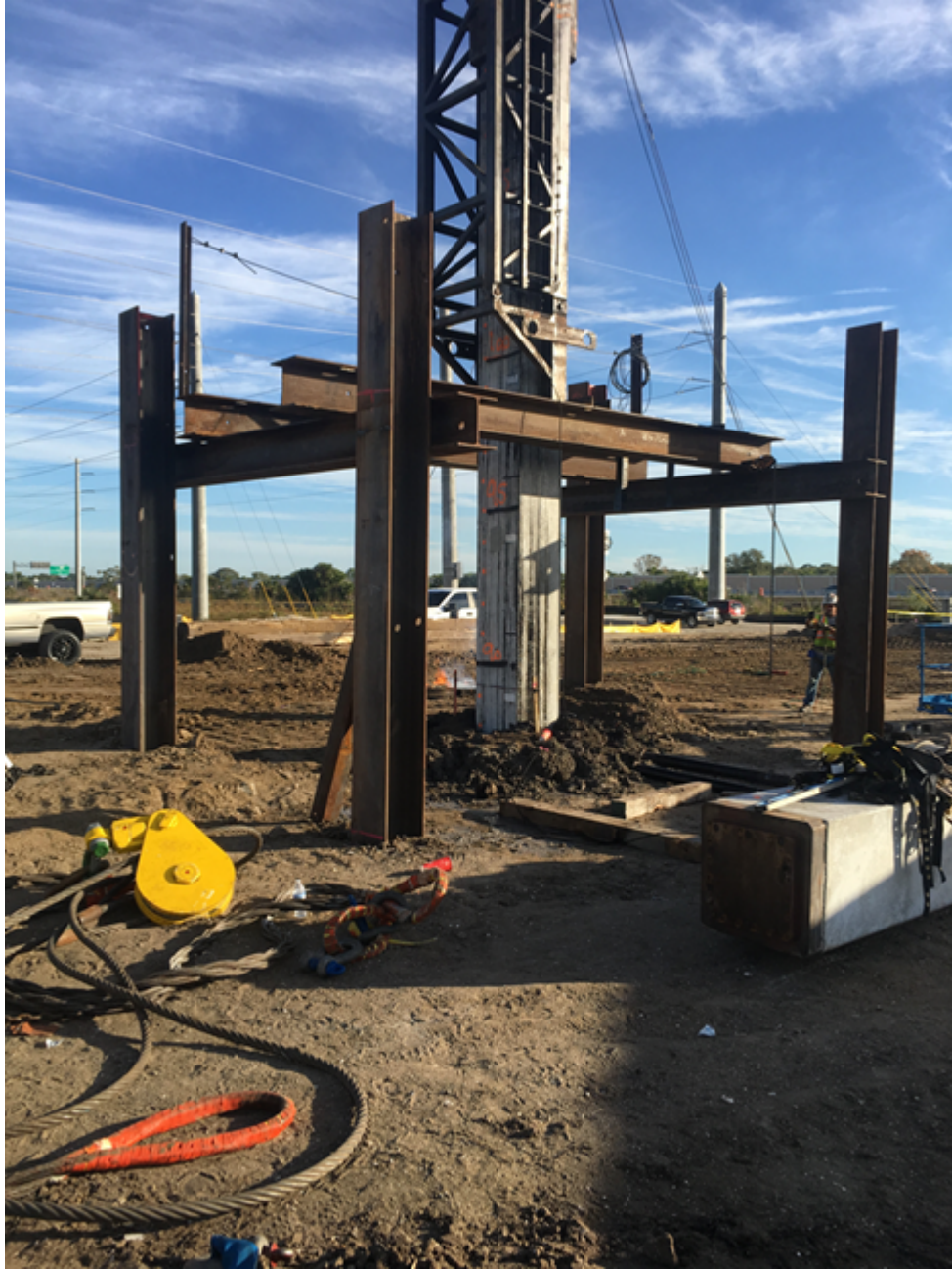
Figure 3-20 Photo of Ellis Road Overpass Test Pile 8 at Bent 1
