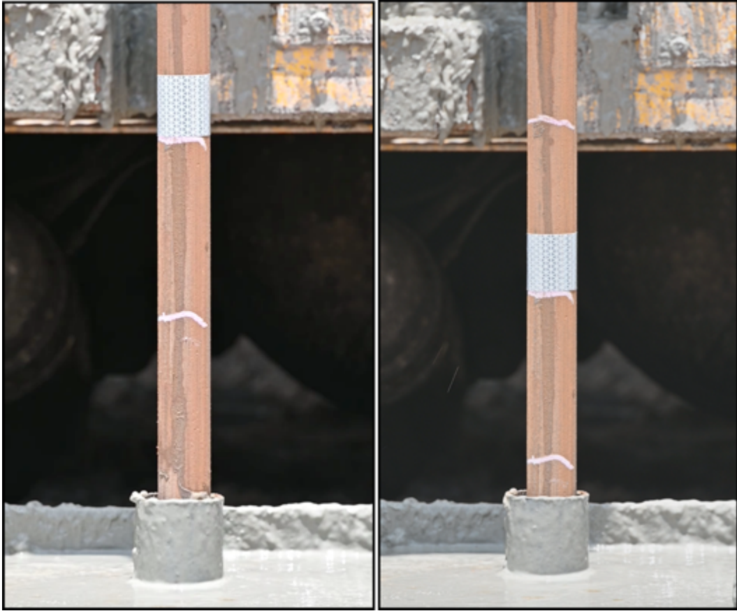
Figure 6-35 CMS and PDM Markings Used for Rod Displacement Monitoring at the Wekiva test site
