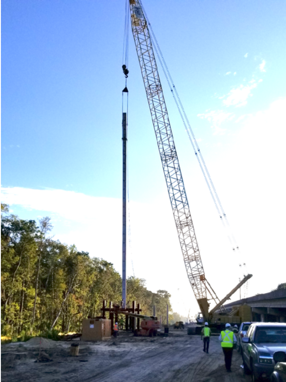
Figure 6-7 Dunns Creek Pile 10 at Pier 4 Installation
