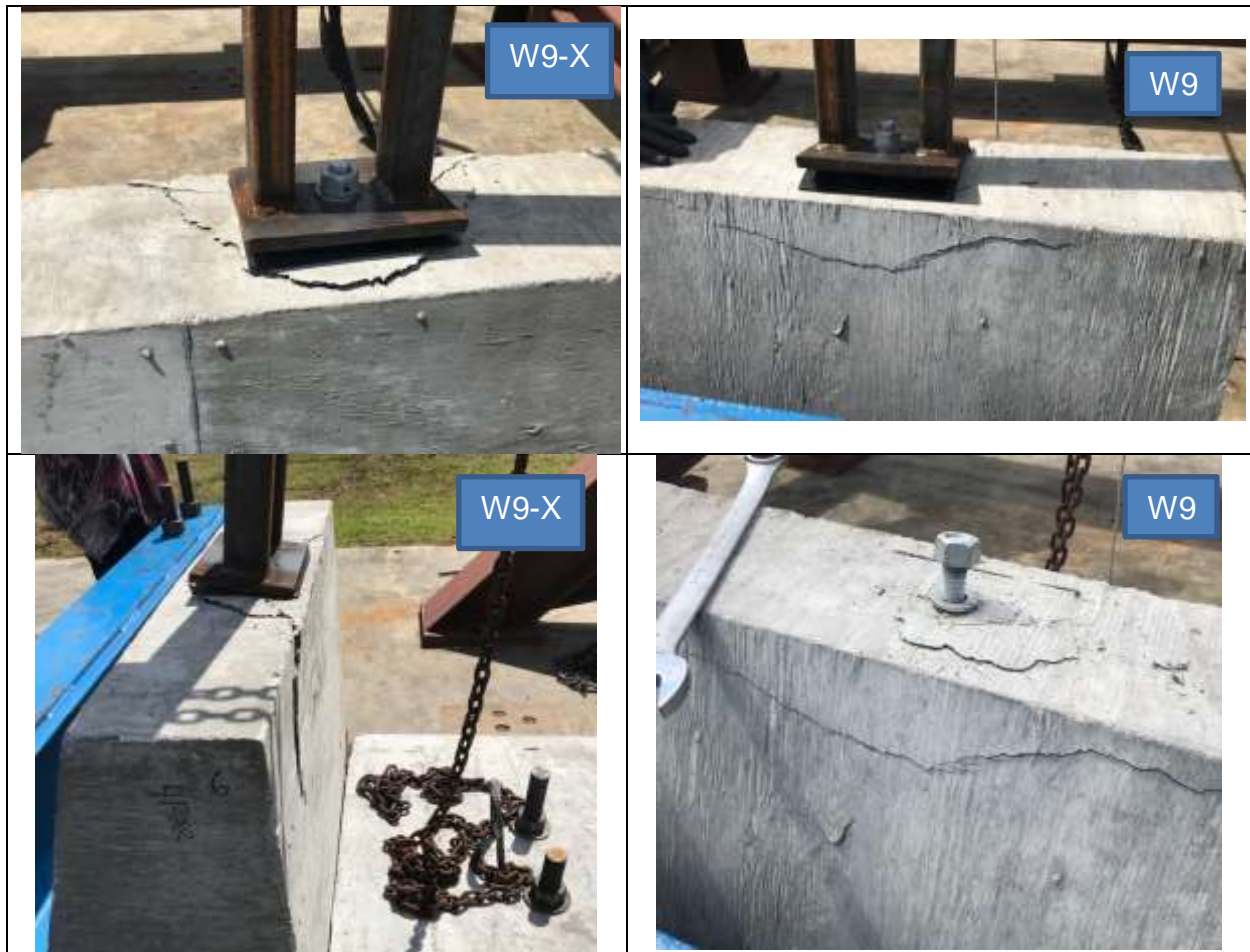
Figure 21: Typical Concrete Breakout Failure Found in Gravity Wall Specimens
