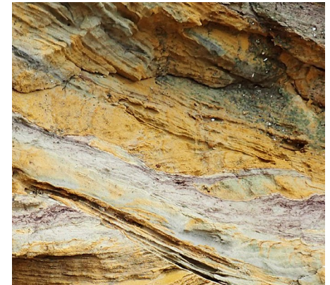
Alum Bluff in NW Florida has complex soil layers that can cause high pile rebound.
