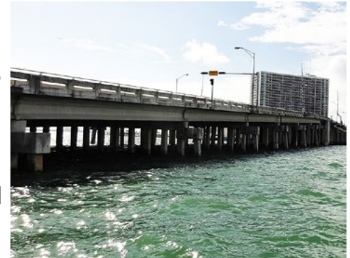
This bridge over Biscayne Bay is one of many transportation structures in Florida founded on driven piles.
