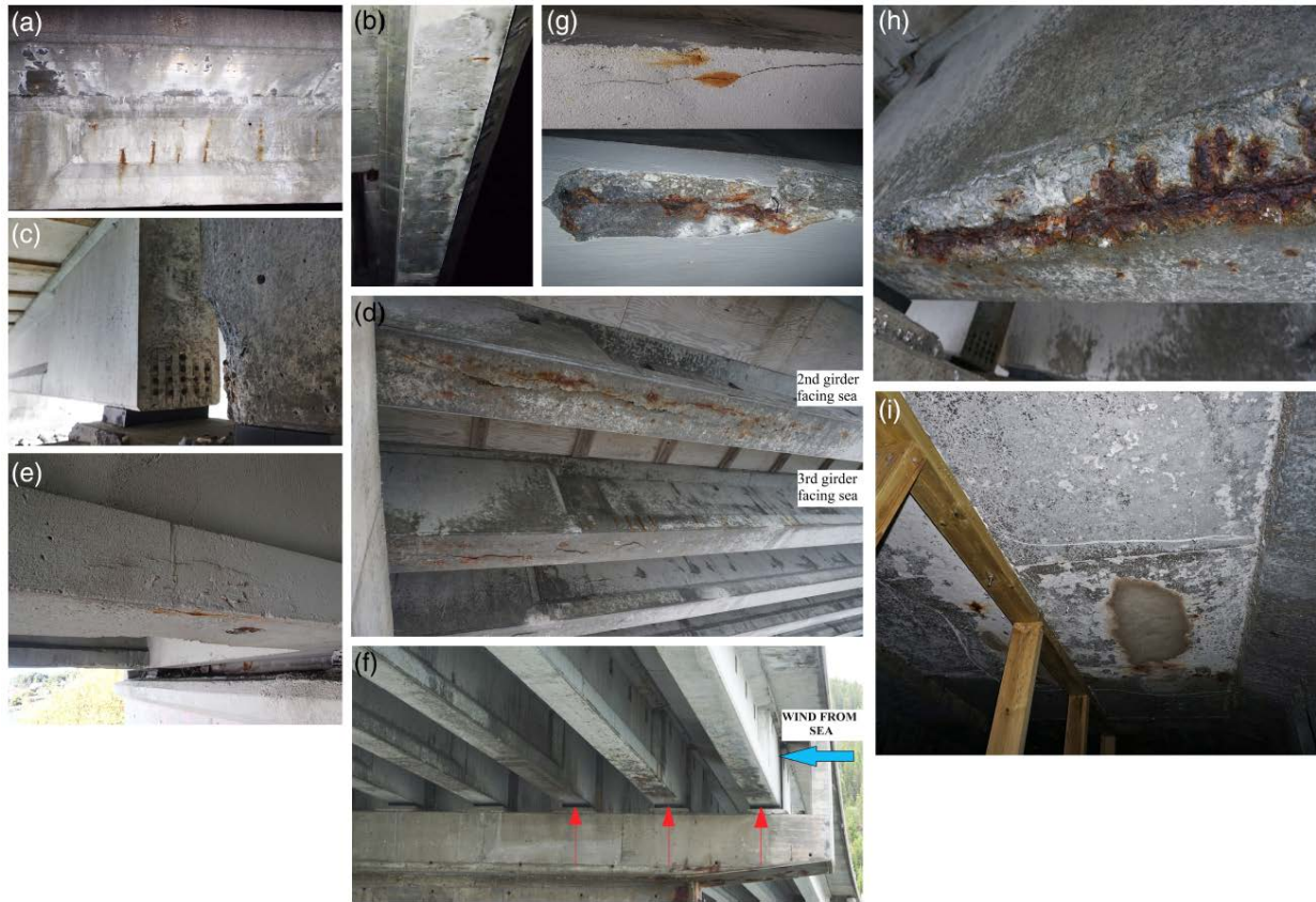
Figure 8. Typical damage reported by Osmolska et al. [1]
