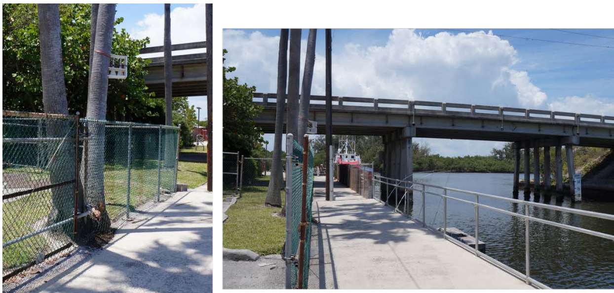
Figure 19. Pictures of the wet candle setup next to bridge #860160. Left closer view of the setup, right with bridge in the image
