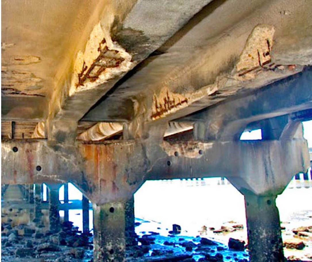
Figure 1. Hornibrook approach bridge; south-facing underside of the bridge [3]
