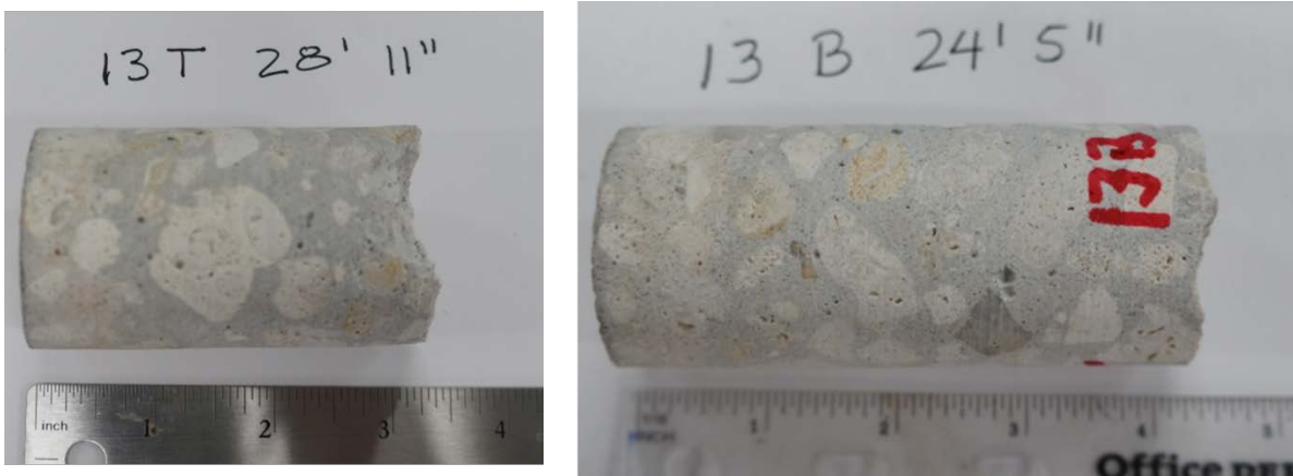
Figure 93. Bent 13 east column east face, Bridge #880005.
