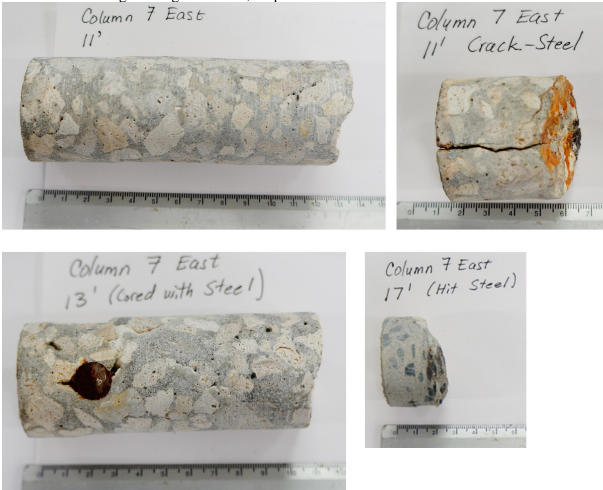
Figure 87. Bent 7 east column east face, Bridge #880005.
