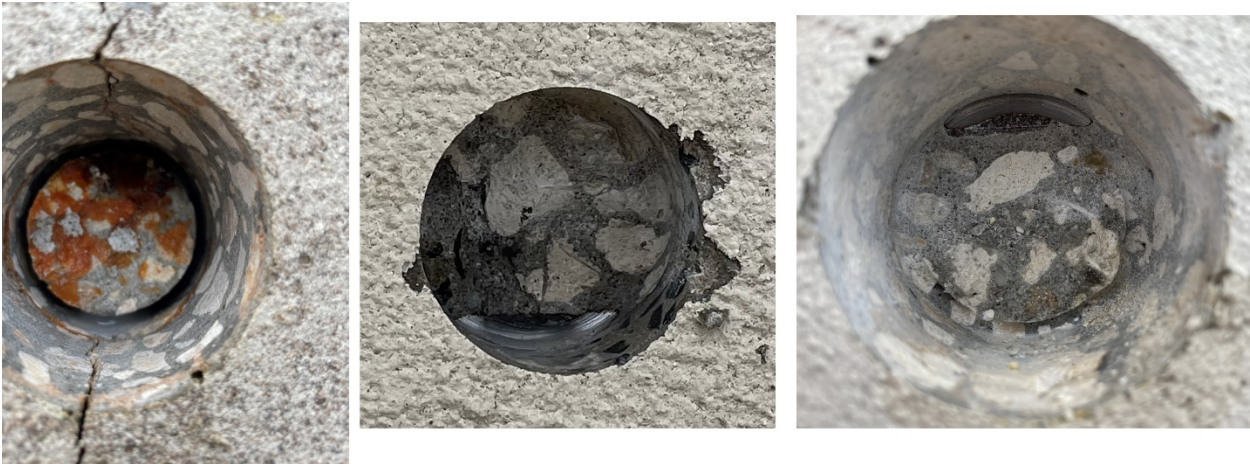
Figure 61. Pictures after removing cores in bent 7.
