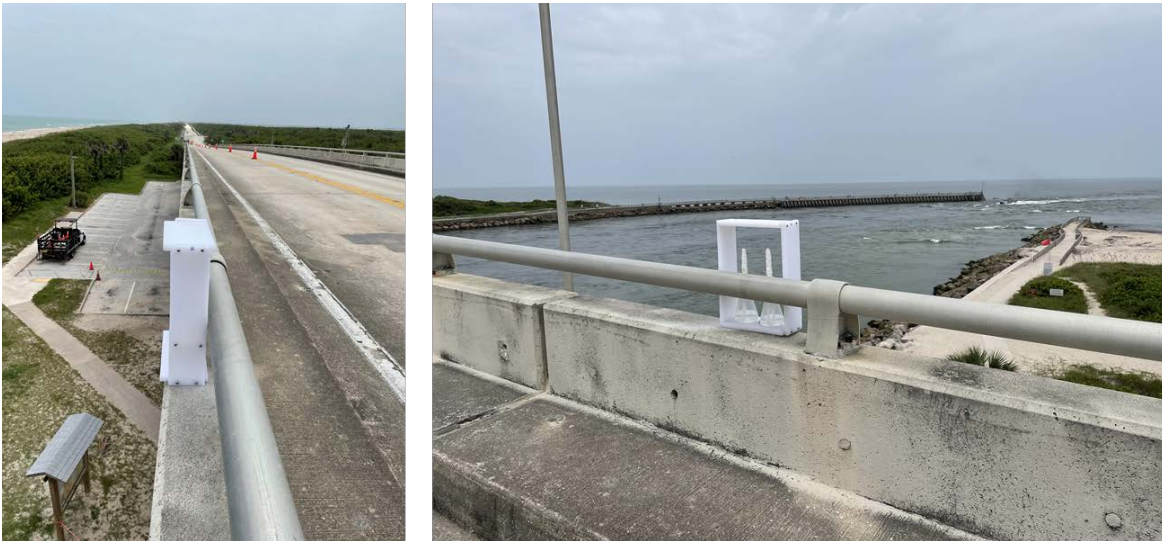
Figure 17. Wet candle setup installed on the top rail of the bridge (Eastward facing)
