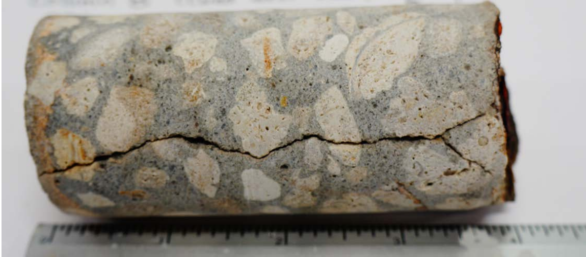
Figure 68. Core obtained bent 8 west column at 22 ft above MHWL
