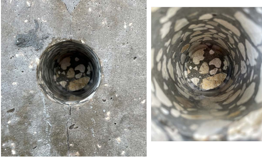
Figure 66. Bridge #100585, images taken after removing core obtained about 5 ft above MHWL, crack was only close to the surface.
