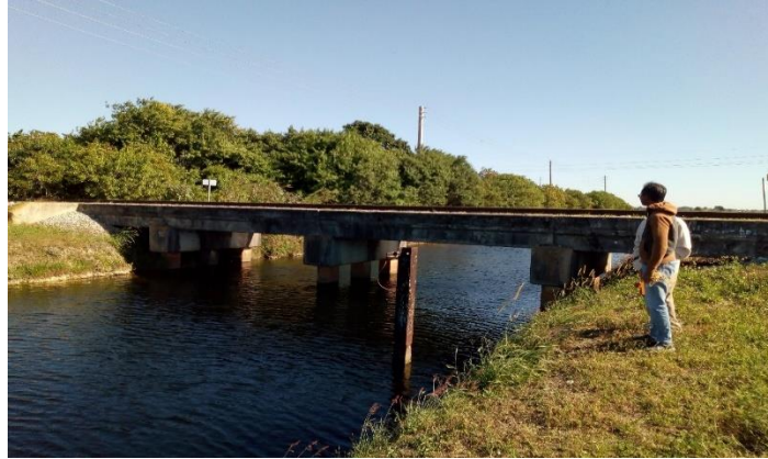
FIGURE 5-2. View of railroad bridge – SXG59.70
