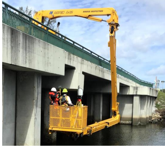
FIGURE 5-9. Field data collection setup with snooper truck
