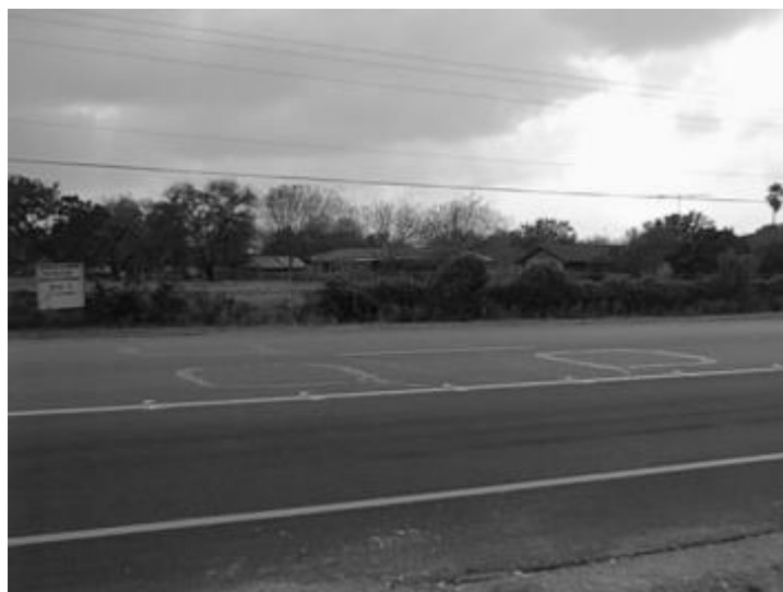
Figure 3-8. Installed Loop Detector (Source: Sunkari et al., 2000)
