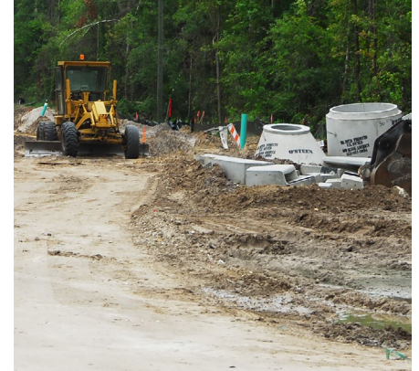
Cast concrete pipe awaits installation at a Florida construction site.
