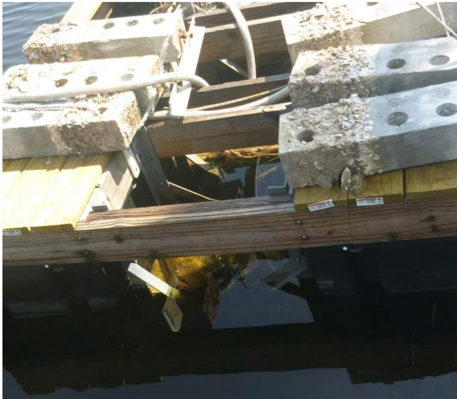
Figure 21. Barge with beams already deployed and fully immersed.
