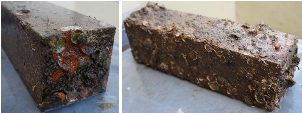
Figure 52. Beams with marine growth.
