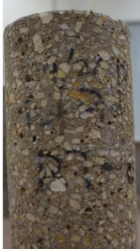
Figure 135. Visual inspection after-split tensile tests on cores of mix 2
