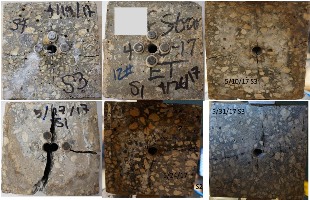
Figure 89. Two- and three-inch-thick samples after MIDT testing.
