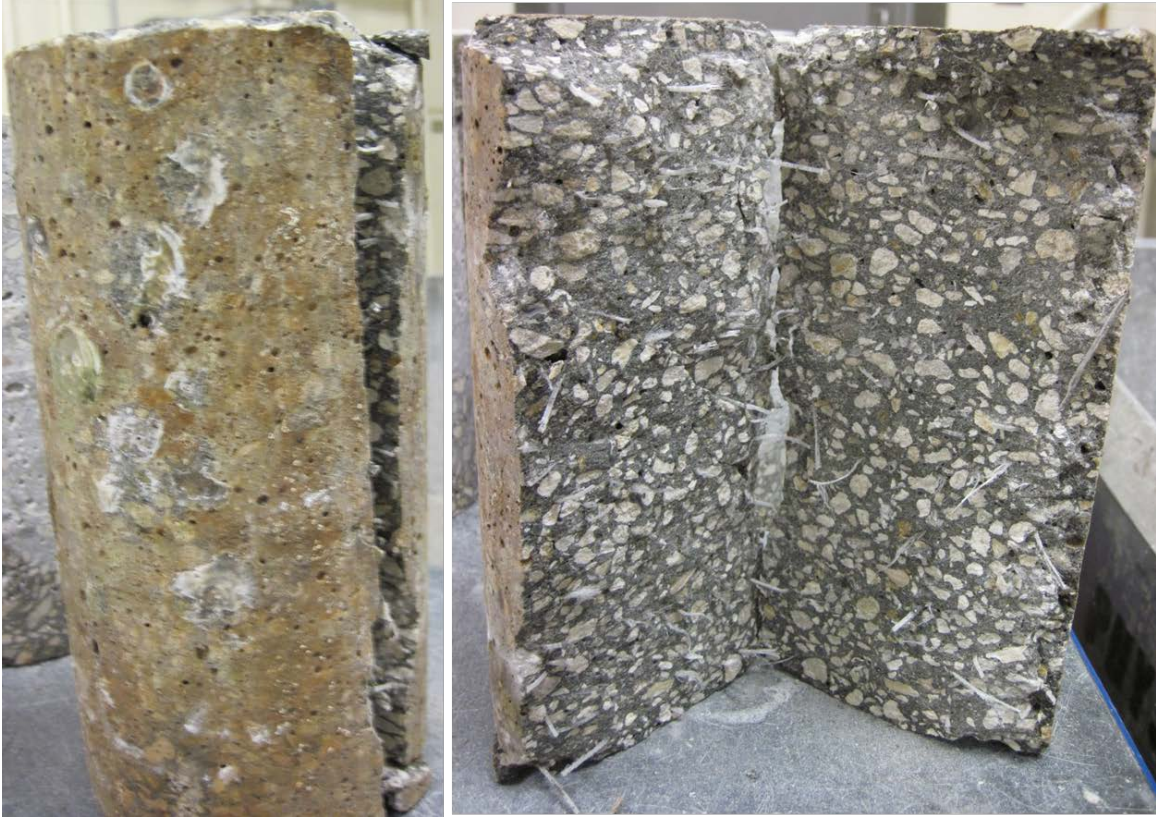
Figure 61. Mix 1 sample (exposed at the barge) after additional hammering.
