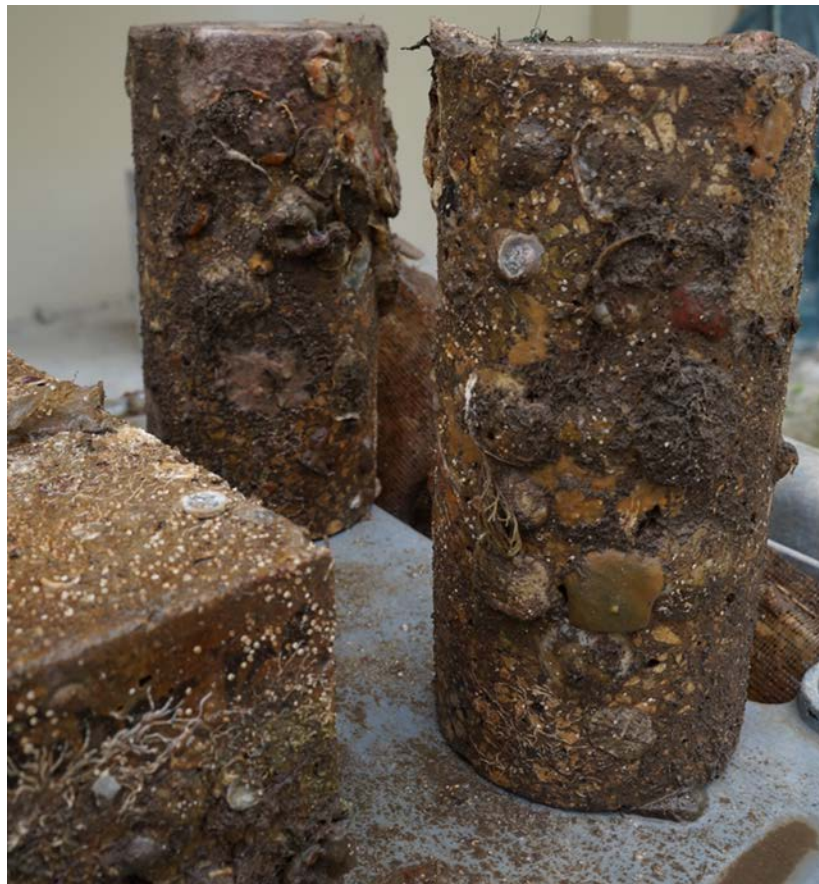
Figure 56. Concrete cores with marine growth
