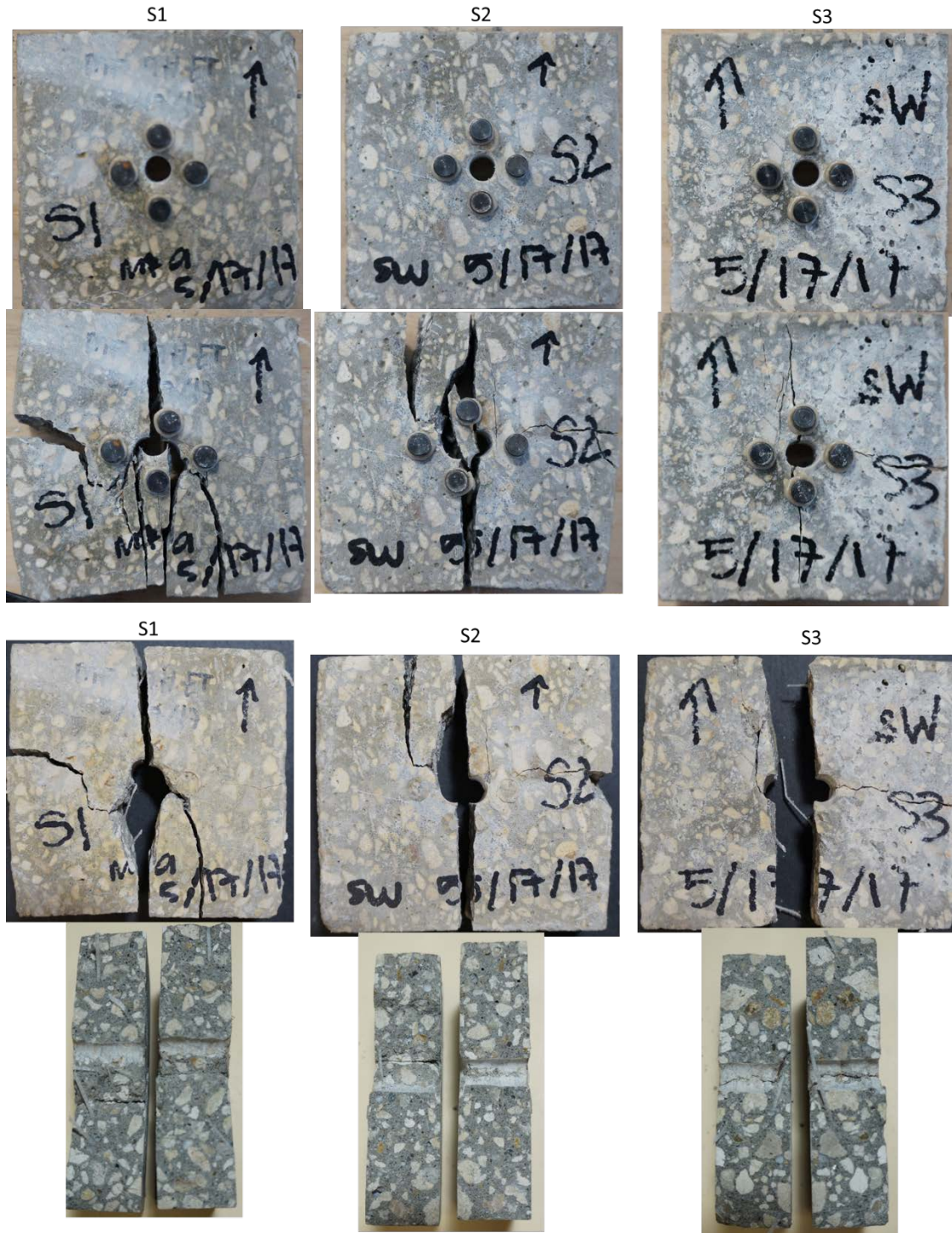
Figure 189. Visual inspection after modified IDT on mix 4 samples (SW)
