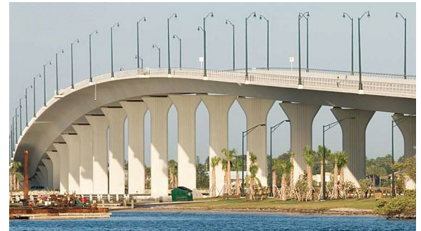
The sinuous Lyons Bridge in Stuart, FL, is a segmental bridge that relies on post-tensioning cables.
