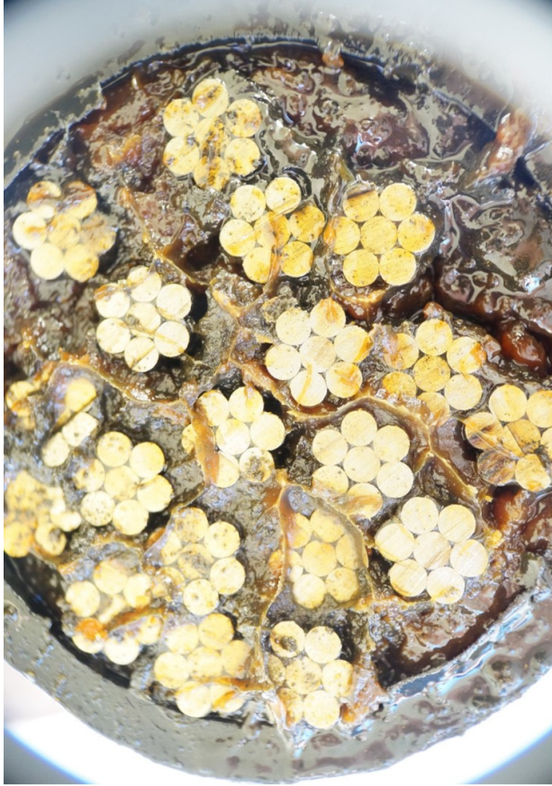
Not Sprayed – Bottom Side
