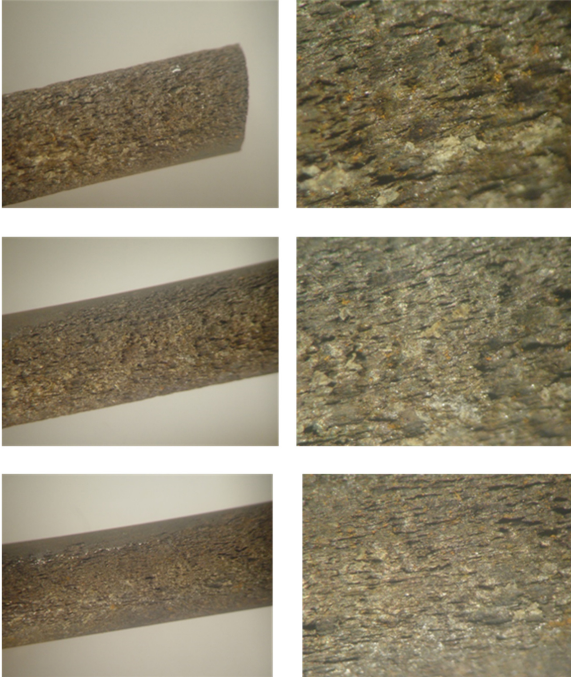
Figure 179. View of 1st strand segment, wire 2 after removing filler and cleaning (close-up 3)
