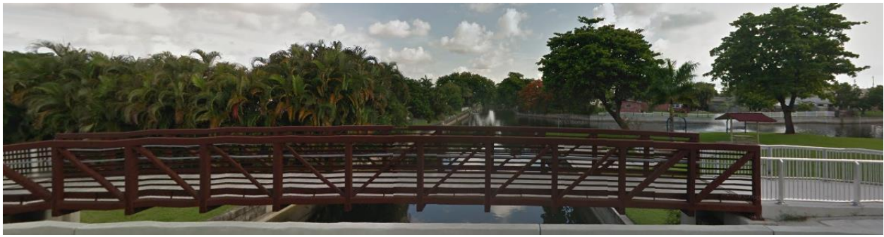
Figure 17: Weathering steel bridge in Margate, FL.
