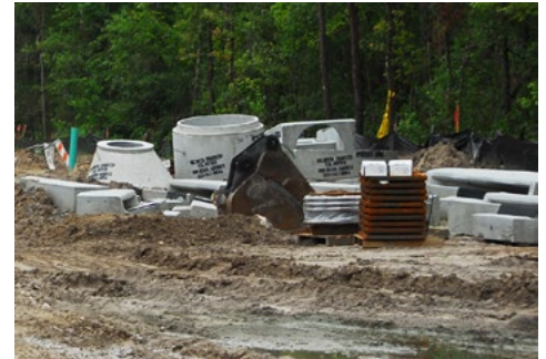
Reinforced concrete stormwater components await installation.
