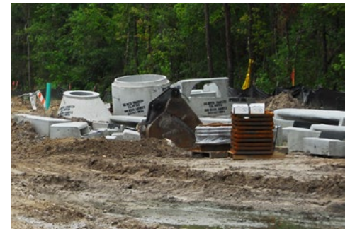
Reinforced concrete stormwater components await installation.
