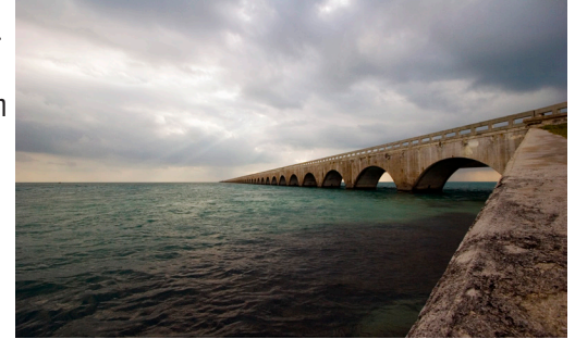
An FDOT research team is investigating the use of hot dipped galvanized steel rebar (HDGR) in the marine splash zone of Florida structures such as bridges.
