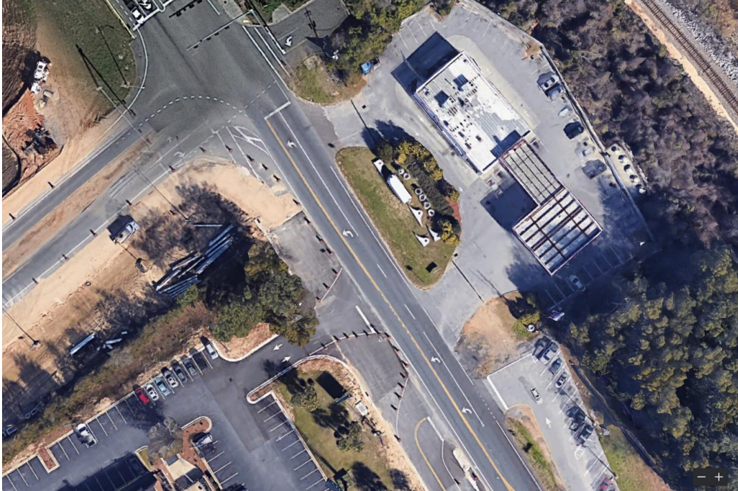
Figure 70. Commercial driveways south of I-10 interchange ramps before reconstruction.
