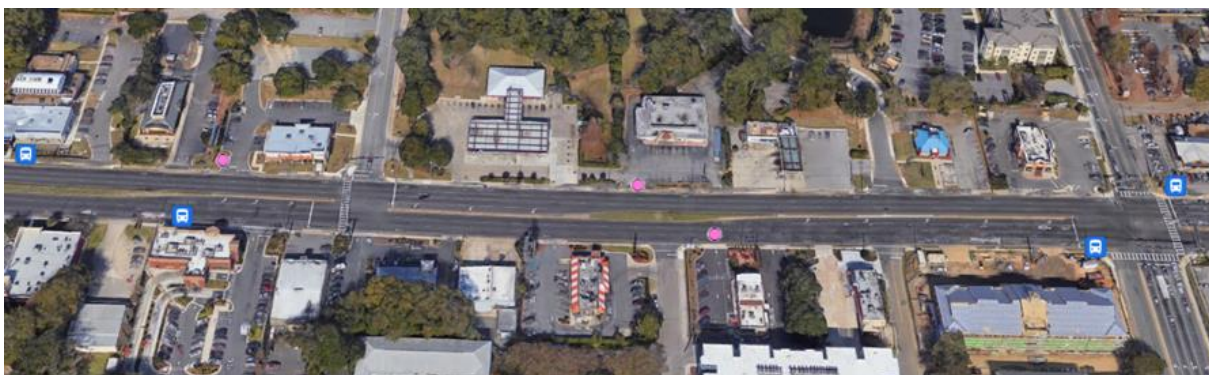
Figure 43. Bicycle and pedestrian crashes on W. Tennessee Street.
