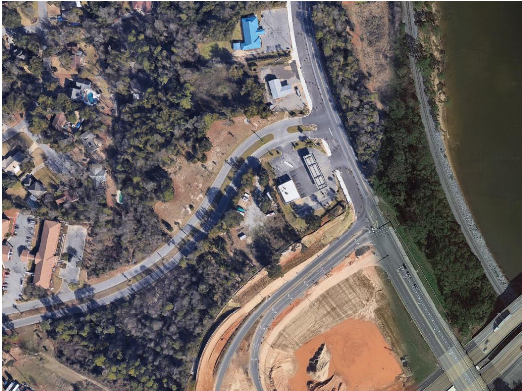
Figure 71. Commercial driveways north of I-10 interchange ramps before reconstruction.
