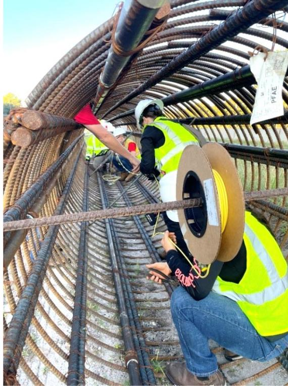
Figure 3.17 Installation of center thermal wire in OC-13 reinforcement cage.
