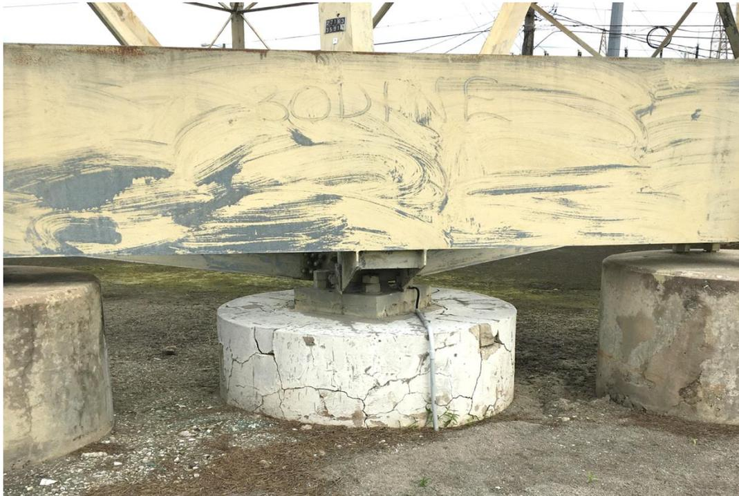
Figure 1.1 Example of a damaged drilled shaft.
