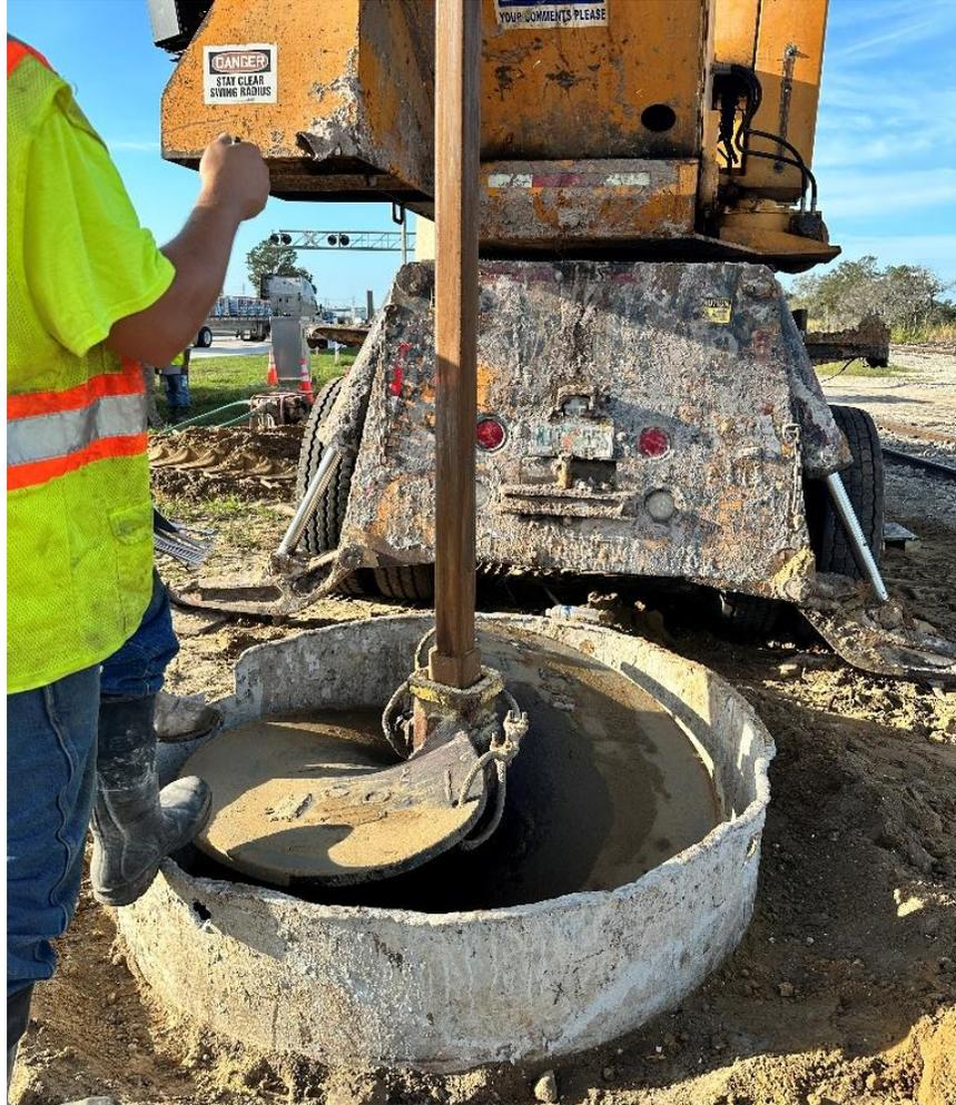
Figure 3.56 Partially augered location of Bartow shaft 1-4 with partial-length casing installed. *[This is a photo showing the construction location of the Bartow drilled shaft. The location is still in the process of being augered. The partial-length casing is already placed inside the augered portion.]*
