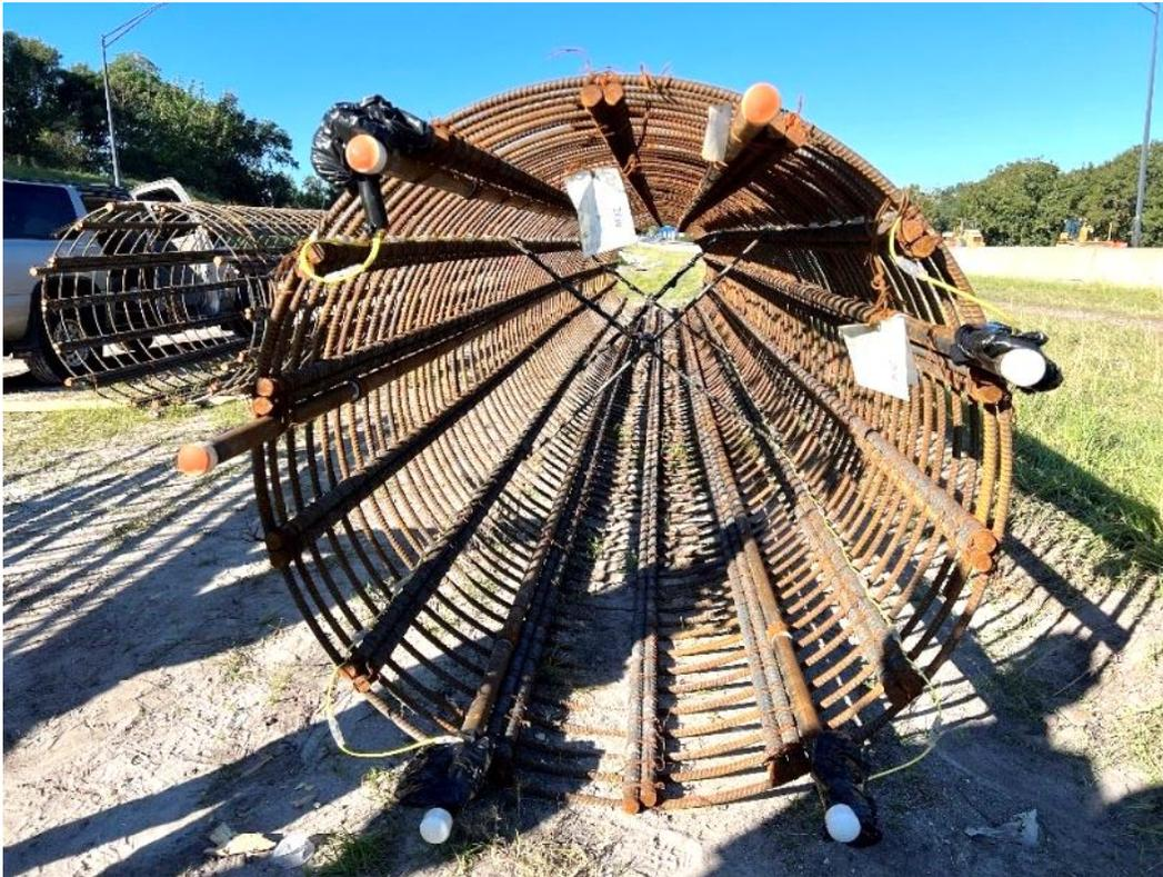
Figure 3.19 Fully instrumented OC-13 reinforcement cage ready to be placed for concrete casting. *[This is a photo taken from outside the top of the OC-13 reinforcement cage. All cage thermal wires and center thermal wire have been installed, and all above-concrete sensors and wire connector ends have been bundled and secured in heavy-duty plastic bags and Gorilla tape.]*
