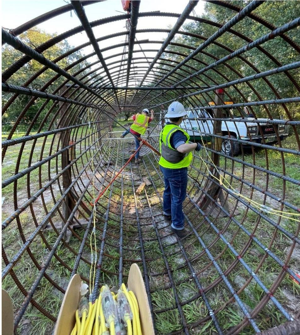
Figure 3.46 Installation of thermal wires along the length of the Sinclair Hills drilled shaft reinforcement cage.
