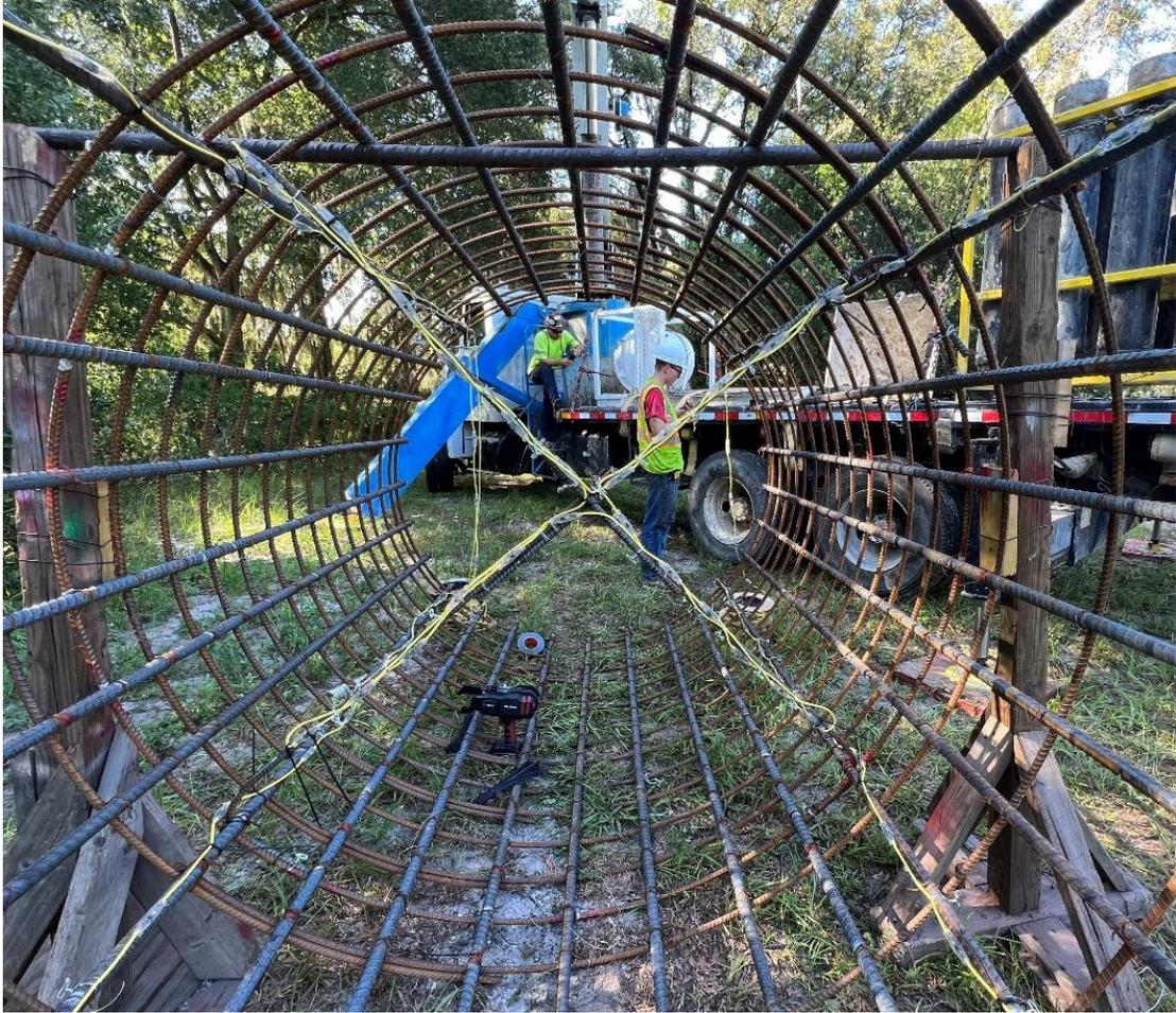
Figure 3.48 Complete installation of center thermal wire inside Sinclair Hills drilled shaft reinforcement cage.
