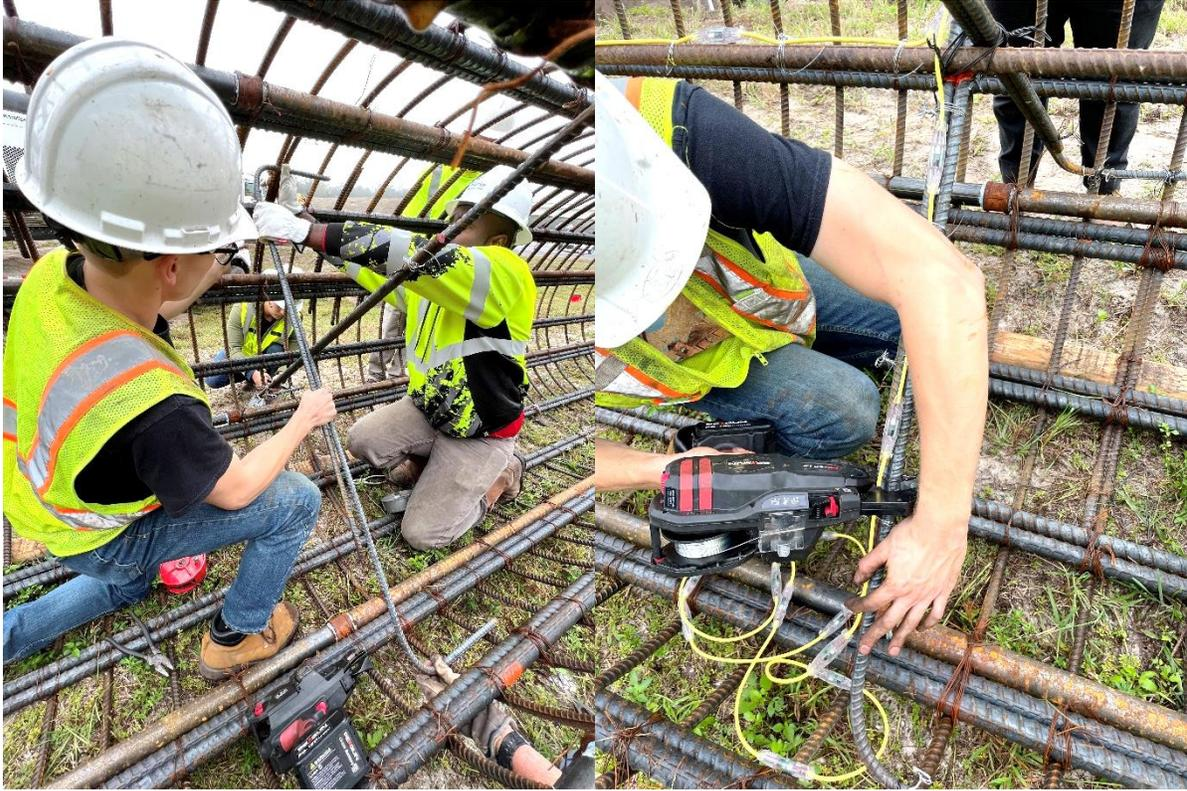
Figure 3.30 Installation of the center rebar cross bracing and the bottom 15 sensors of the center thermal wire in an across-shaft configuration along the bottom rebar cross bracing in OC-19 reinforcement cage.
