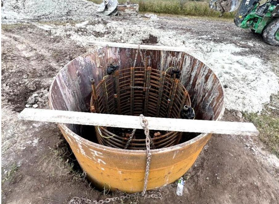
Figure 3.20 Fully instrumented OC-13 reinforcement cage placed in the augered location prior to concrete placement.
