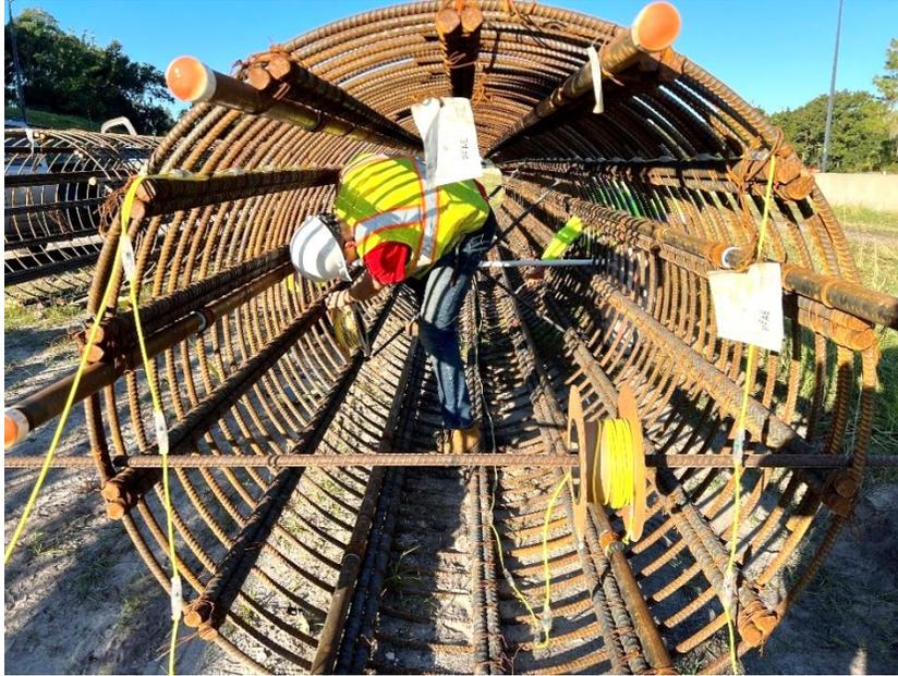
Figure 3.15 Installation of thermal wires along the length of the OC-13 reinforcement cage.
