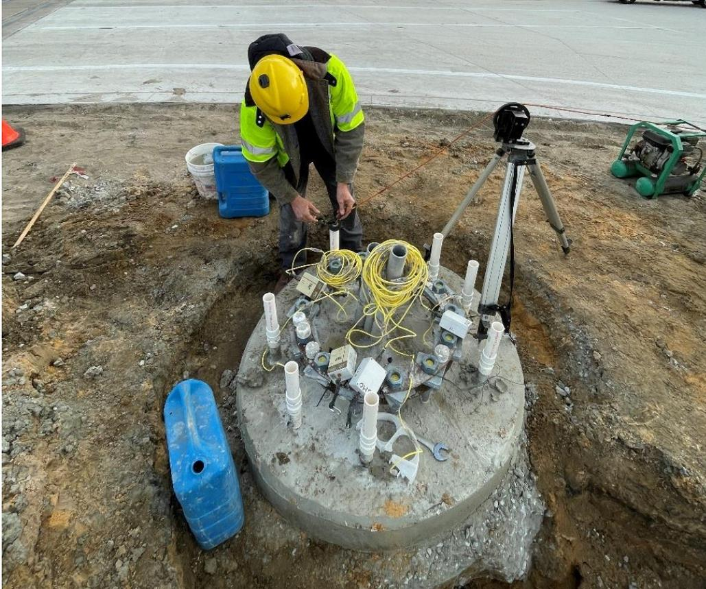
Figure 1.8 TIP probe system in use.
