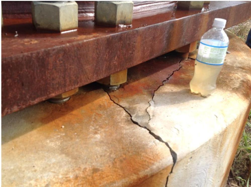
Figure 1.2 Temperature-induced damage to drilled shaft (courtesy of Chris Harris with R.W. Harris, Inc.).
