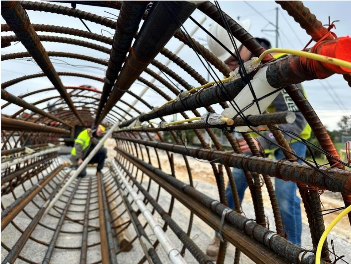
Figure 3.57 Close up view of thermal wire installed at the reinforcement cage with offset return wire.
