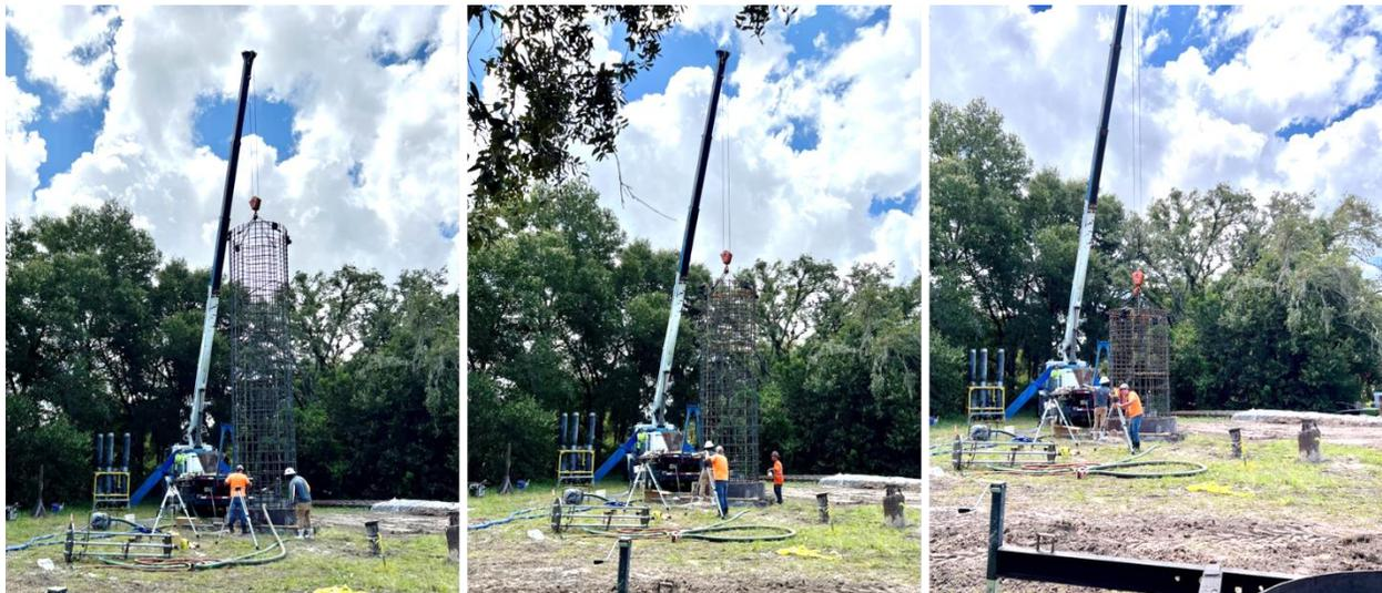
Figure 1.5 Drilled shaft reinforcement cage placement.
