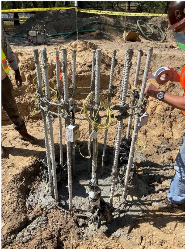
Figure 3.5 Connection of the Thermal Acquisition Port boxes after concrete placement. *[This is a photo of DS-6 after concrete placement with approximately five feet of rebar stick-up illustrating the connection of Thermal Acquisition Port boxes to the thermal wires to begin data collection.]*
