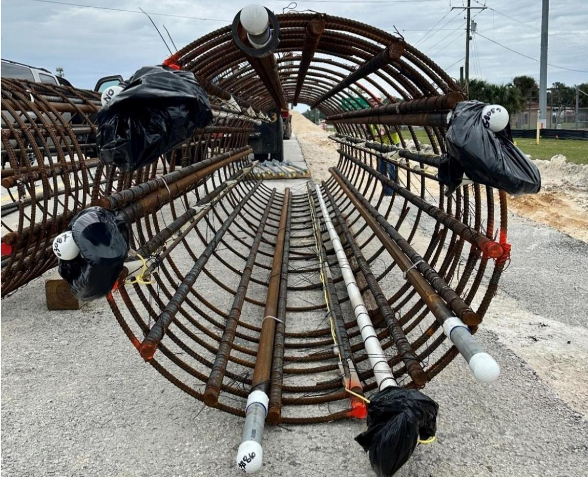
Figure 3.58 Fully instrumented Bartow shaft 1-4 reinforcement cage ready to be placed for concrete casting.
