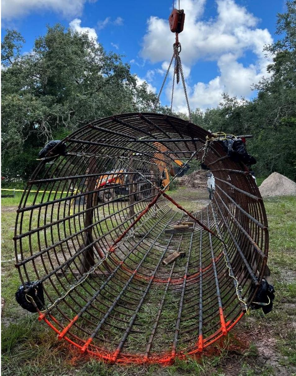
Figure 3.49 Fully instrumented Sinclair Hills drilled shaft reinforcement cage ready to be placed for concrete casting.
