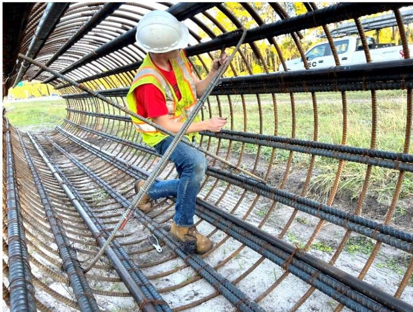
Figure 3.16 Installation of the center rebar cross bracing for drilled shaft OC-13.
