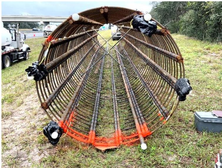
Figure 3.32 Fully instrumented OC-19 reinforcement cage ready to be placed for concrete casting.
