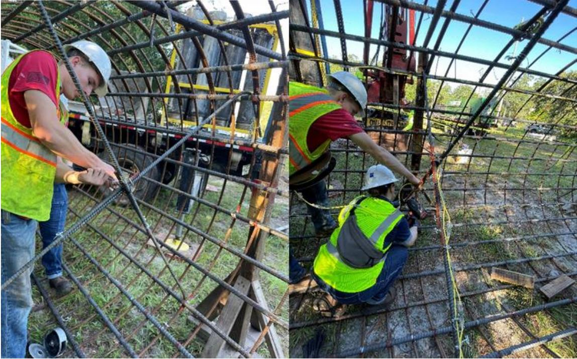
Figure 3.47 Installation of the rebar cross bracing and the center thermal wire in an across-shaft configuration along the rebar cross bracing.
