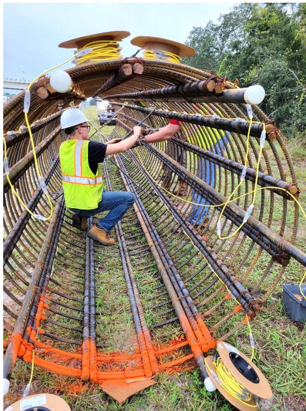
Figure 3.29 Installation of thermal wires along the length of the OC-19 reinforcement cage. *[This is a photo taken from the top of the OC-19 reinforcement cage showing installed cage thermal wires positioned roughly 90 degrees apart radially.]*
