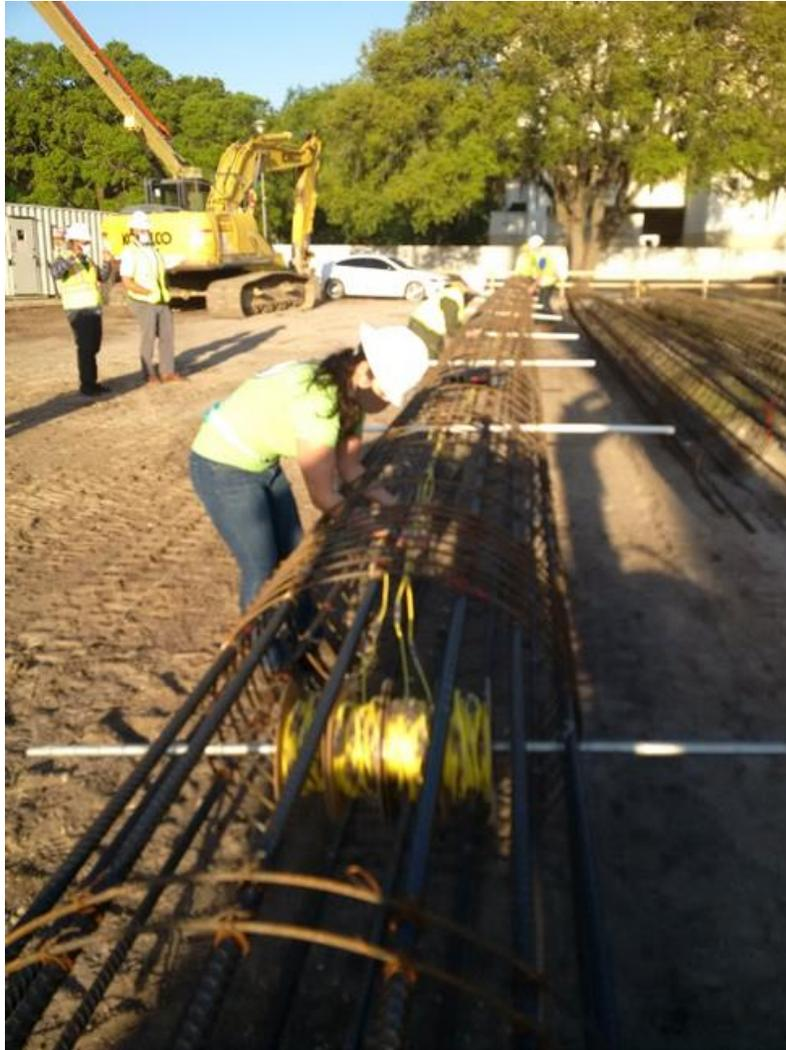
Figure 1.7 Installation of thermal wires to a shaft reinforcing cage at a construction site located on the University of South Florida Tampa Campus.
