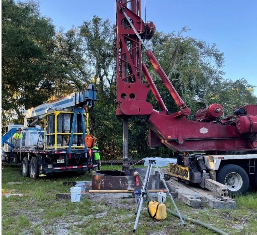
Figure 3.45 Excavation of the Sinclair Hills drilled shaft with partial-length casing installed. *[This is a photo showing the construction location of the Sinclair Hills drilled shaft. The location is still in the process of being augered with slurry flowing from a large hose line. The partial-length casing is already placed inside the augered portion.]*
