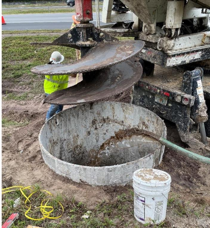
Figure 3.28 Excavation of drilled shaft OC-19 with partial-length casing installed.
