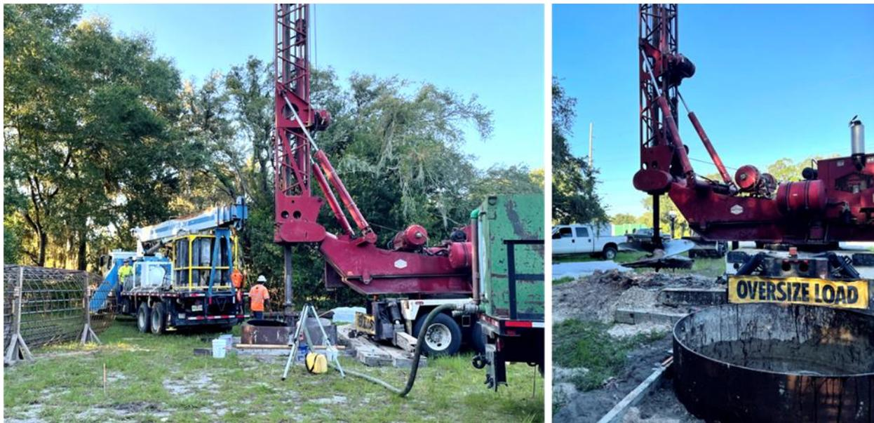
Figure 1.4 Drilled shaft excavation.
