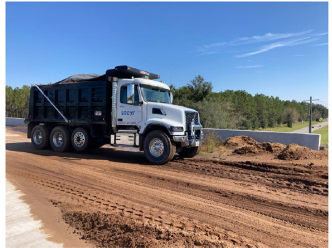
A 70-kip loaded truck is parked over a pile in end bent at the Sandridge Road testing site.
