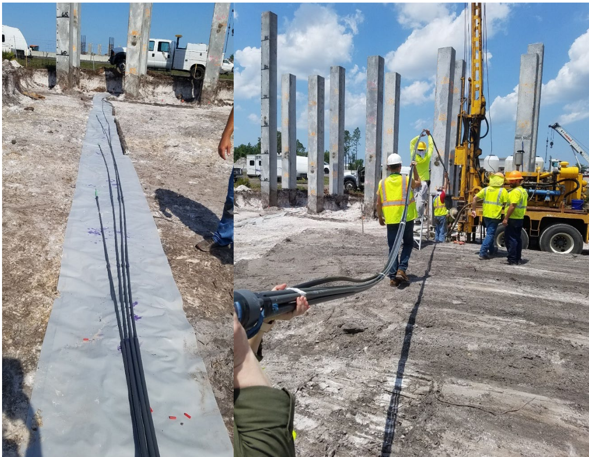
Figure 3.17 Extensometer assembly installation (Paseo Al Mar Blvd).
