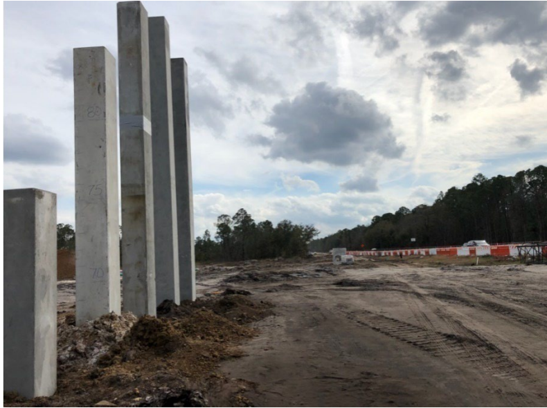
Figure 3.6 End Bent 1 looking south; Pile 3 has duct tape holding lead wires used to protect them during driving (Pile 1 farthest to the south; used with permission from J. Bosnoian, HTNB)
