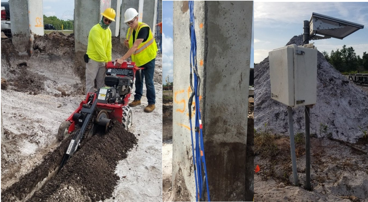
Figure 3.16 Trenching for conduit placement (left), wire splicing (center), and datalogger enclosure (right)
