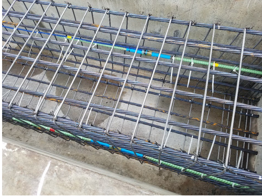
Figure 3.29 Geokon VW rebar strainmeters tied to pile rebar cage (Henley Rd project)
