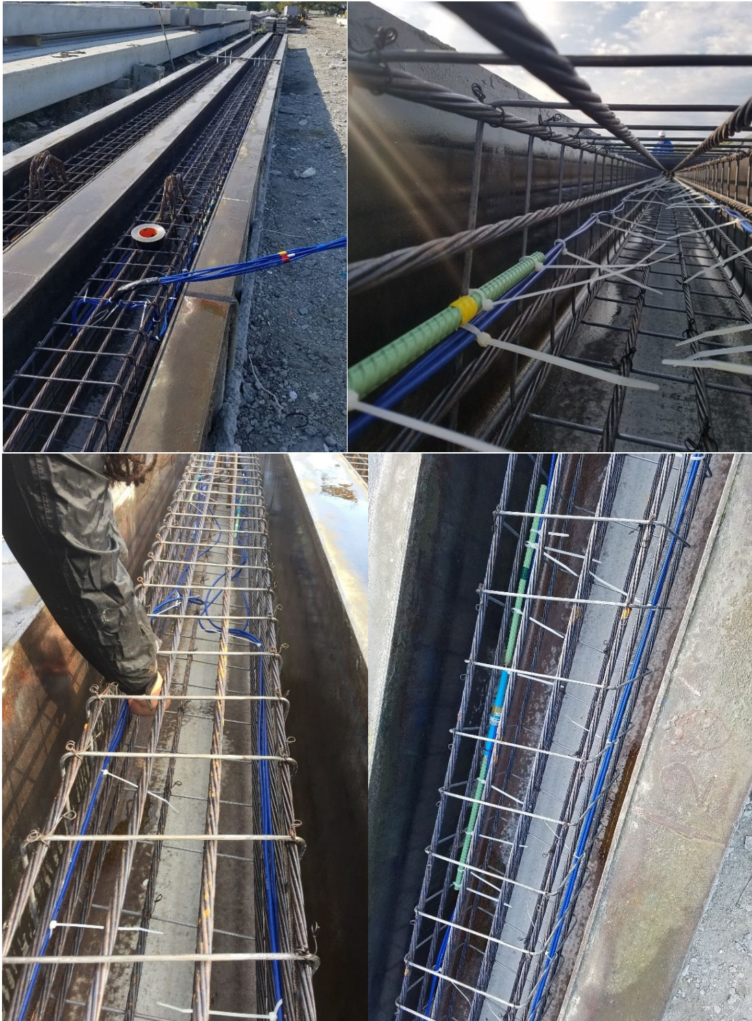
Figure 3.11 Instrumentation of Pile 4 (18 in) for End Bent 1 (Sandridge Road).
