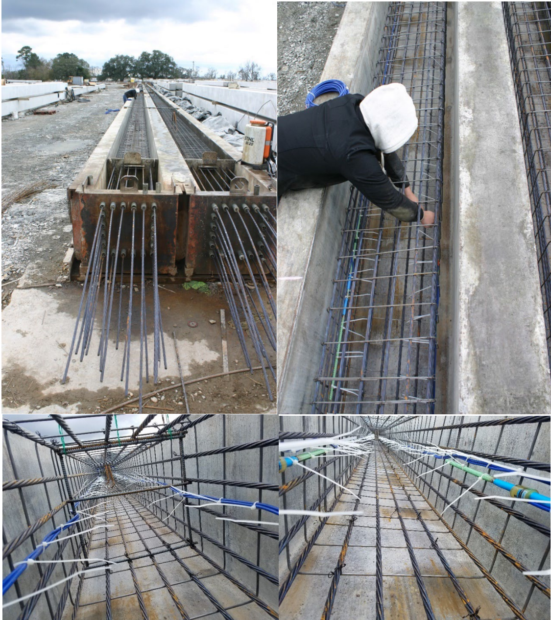
Figure 3.4 Instrumentation of Pile 3 (24 in) for End Bent 1 at Henley Road (Bridge 710120).
