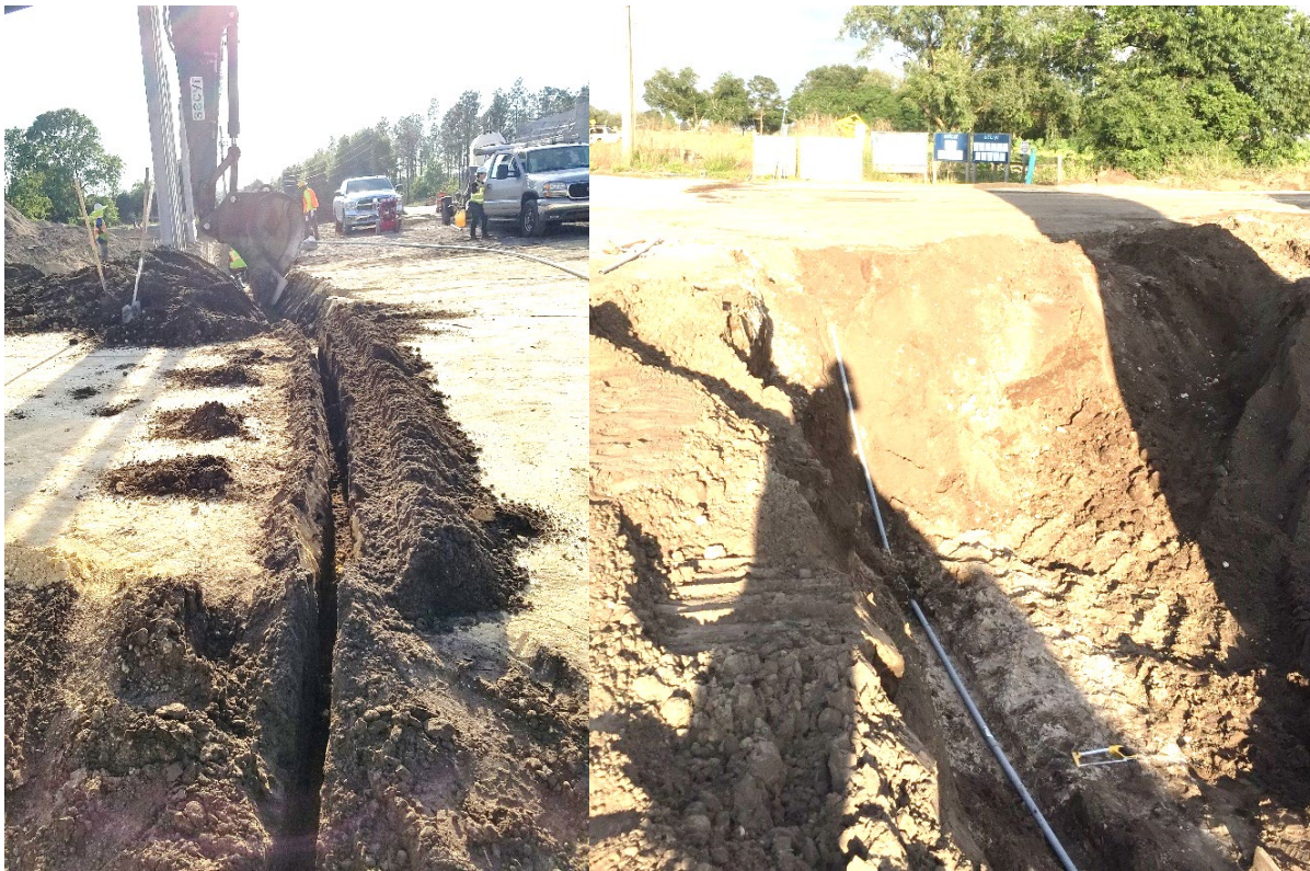
Figure 3.19 Trenching and conduit installation for lead wires (Sandridge Rd).
