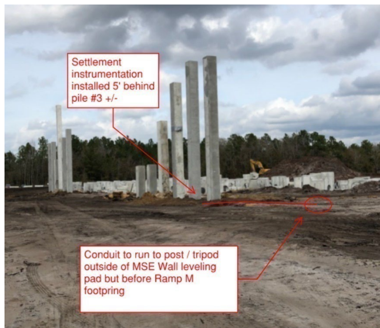
Figure 3.7 End Bent 1 looking north; approximate location of the data collection system outside the embankment footprint (used with permission from J. Bosnoian, HTNB).
