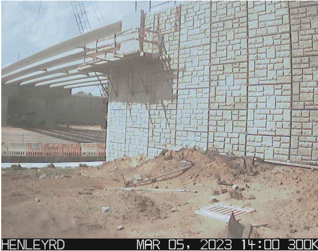
Figure 6.18 Henley Rd bridge with girders but no deck in place
