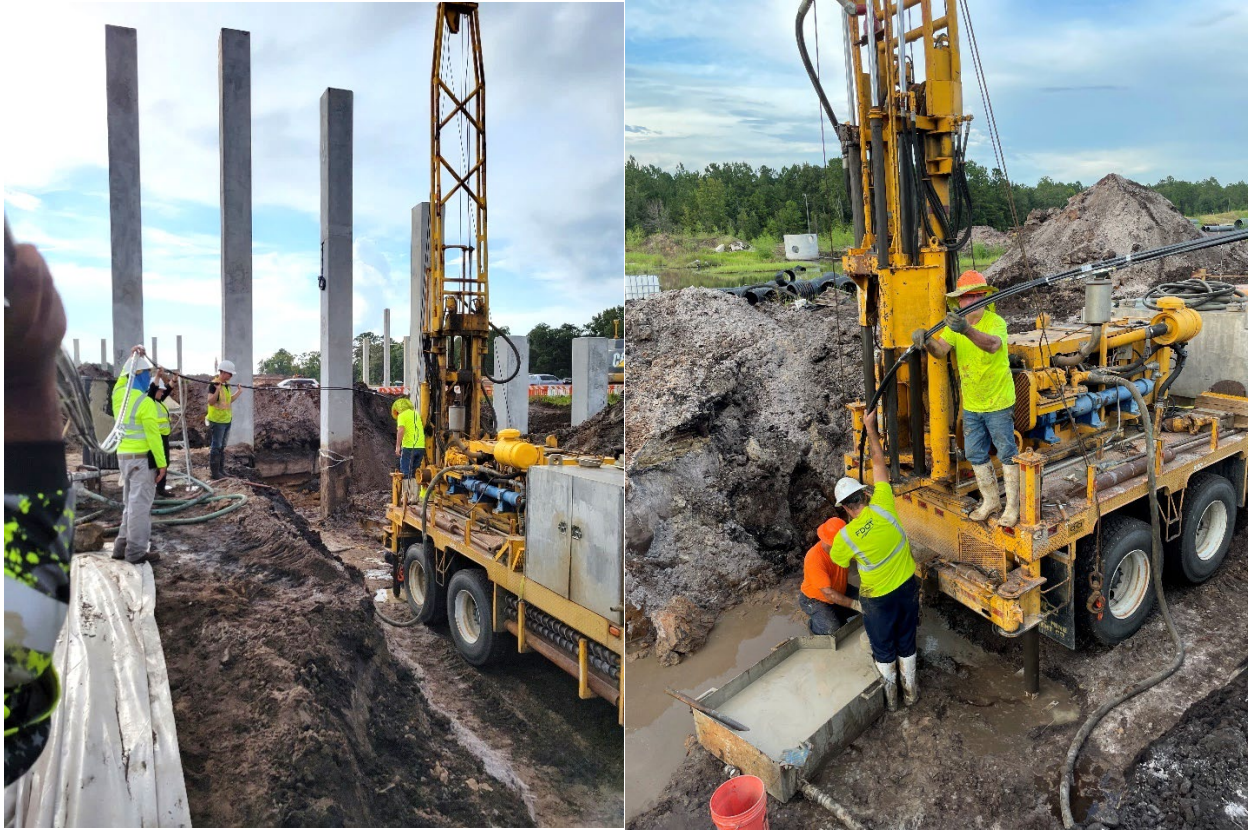
Figure 3.22 Settlement assembly supported and negotiated into borehole by multiple installers.
