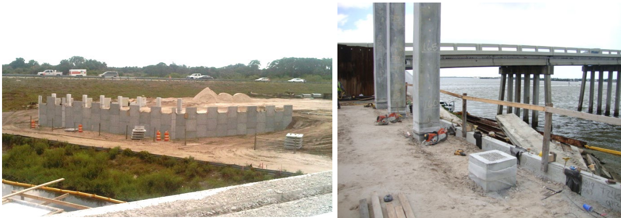
Figure 1.1 Early stages of embankment filling and MSE wall construction (left); final stages behind MSE wall (right).
