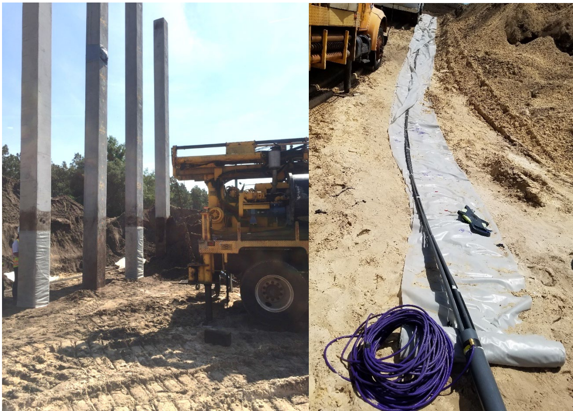
Figure 3.18 Borehole drilling location (left) and extensometer assembly (right) at Sandridge Rd
