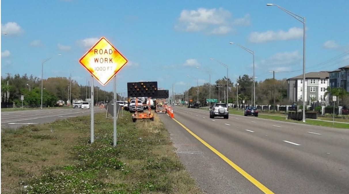
Figure 86. Field View of Construction Zone on US-301
