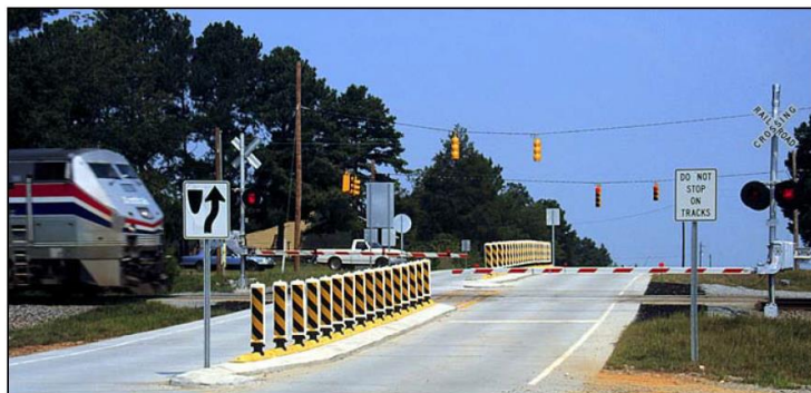
Figure 1-5 Example of Qwick Kurb (Photo courtesy of NCDOT)
