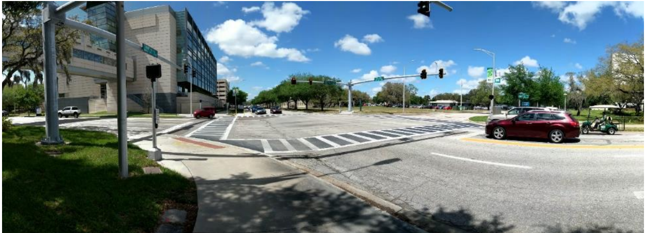
Figure 32. Signalized intersection, USF Tampa campus
