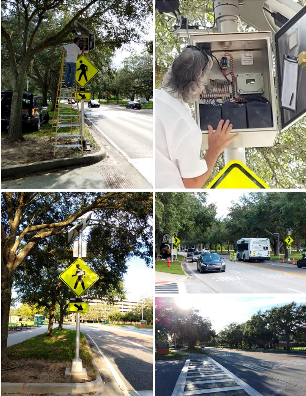
Figure 39. Installation of system at midblock crosswalk in Tampa
