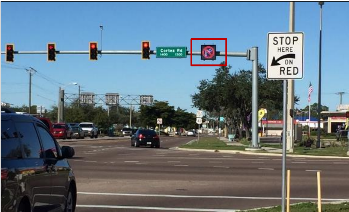
Figure 7. D1 site after implementation of “No Turn on Red” blank-out sign
