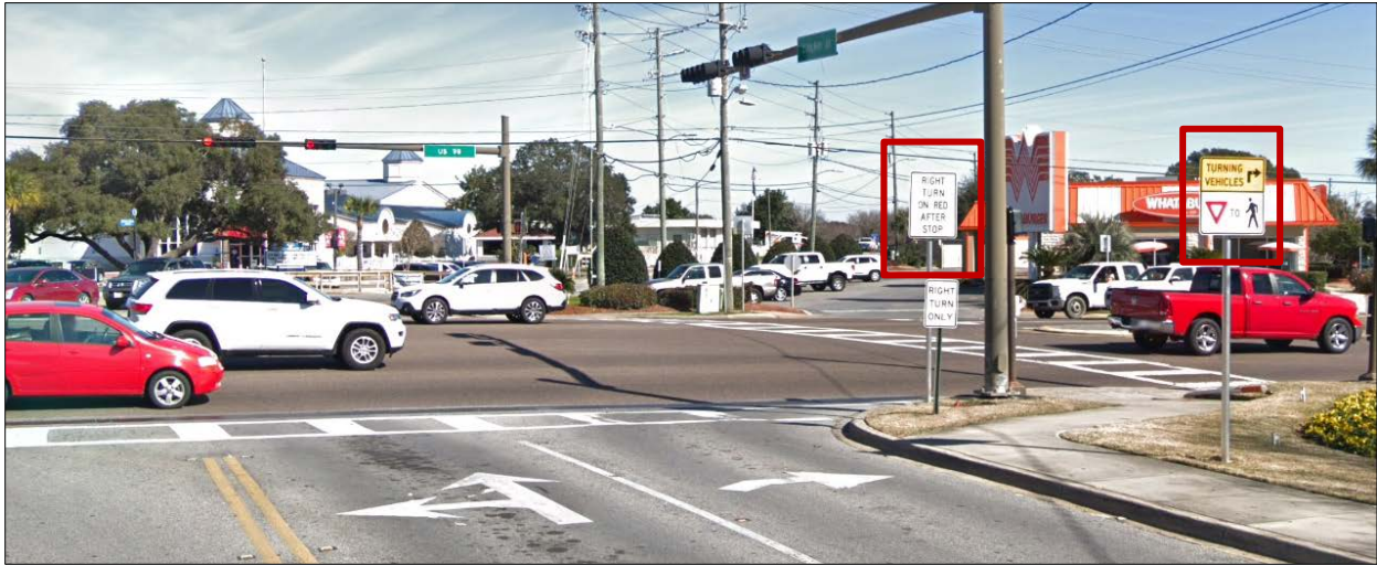
Figure 12. D3 site after implementation (NB) of both “Right on Red After Stop” and “Turning Vehicles Yield to Pedestrians” signs
