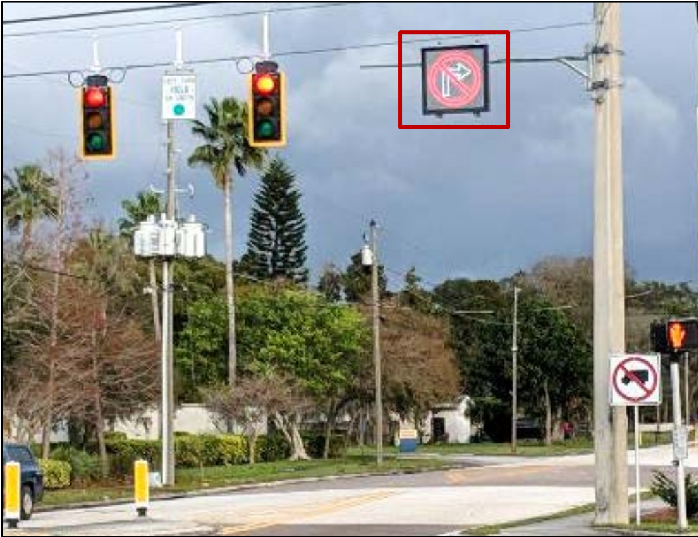
Figure 22. D7 site after implementation of “No Turn on Red” blank-out sign
