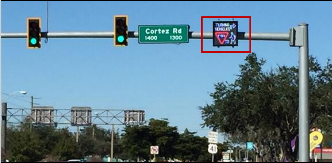
Figure 8. D1 site after implementation of “Turning Vehicles Yield to Pedestrians” blank-out sign
