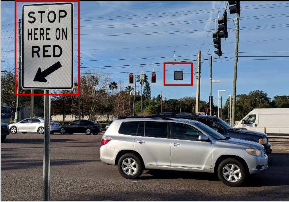
Figure 21. D7 site after implementation of blank-out sign and “Stop Here on Red” sign
