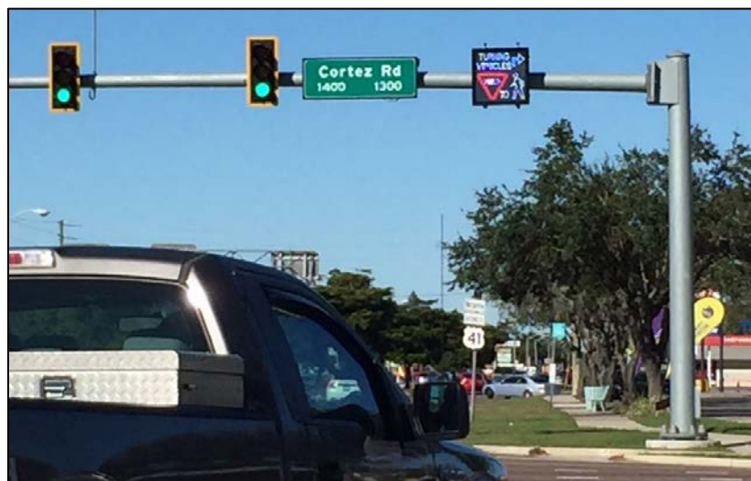
Figure 85. Example of “Turning Vehicles Yield to Pedestrians” blank-out signs
