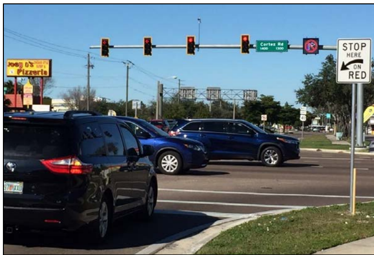
Figure 86. Example of “Stop Here on Red” sign.
