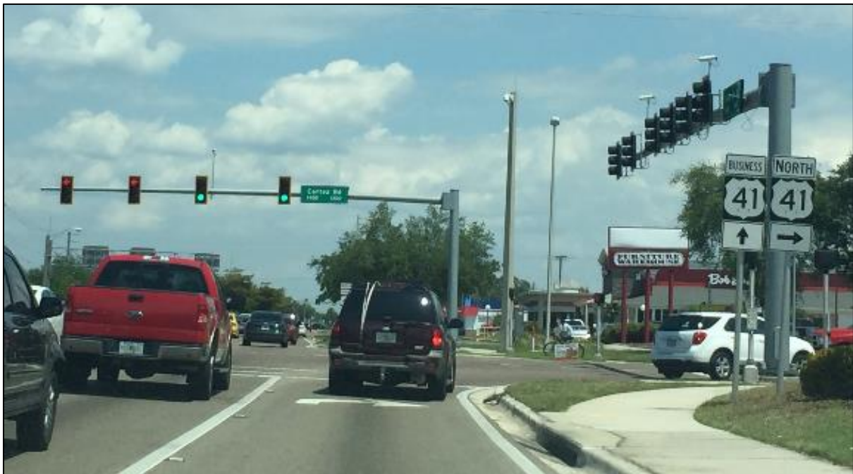
Figure 5. D1 site before implementation
