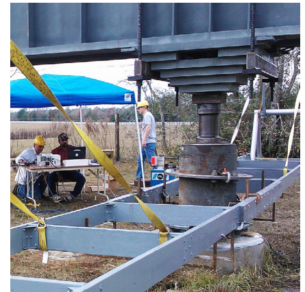
Load testing a drilled shaft piling involves exerting enormous pressures and observing the subtle movements of the drilled shaft.
