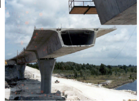
Post-tensioning makes longer, lighter bridge segments possible.
