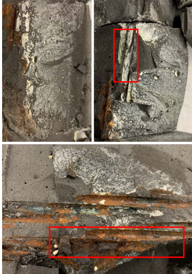
Figure 5-8: Images of the interior pores and voids contained in the 3-ft chloride-contaminated grout with impregnation material.
