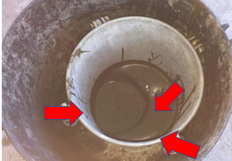
Figure 4-15: The property of thixotropic grout.
