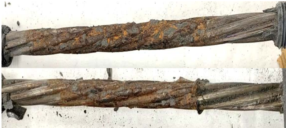
Figure 5-10: An image of the reinforcement extracted for the 1-ft chloride-contaminated tendons. The top image is the control tendon and the bottom image is the impregnated tendon.
