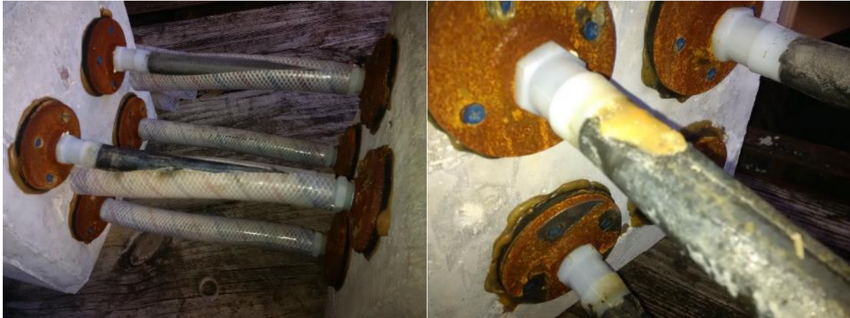
Figure 4-59: Connecting hoses removed showing residual impregnation product.
