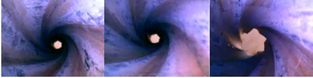
Figure 4-48: Sample 1-1 (none) lowest void perfect grout distribution.
