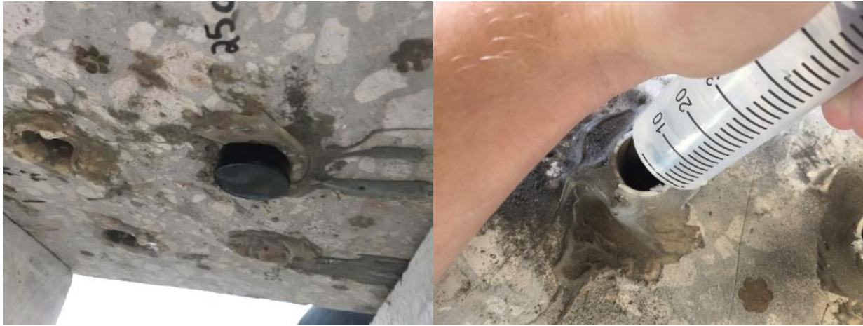
Figure 4-44: Rubber plug installed into the front face of concrete specimen 1 (left); water injection into vacated duct (right).
