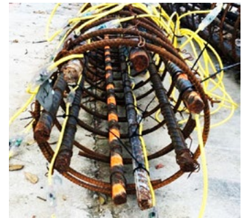
Steel reinforcing cage wired with temperature sensors before placement in concrete pile.
