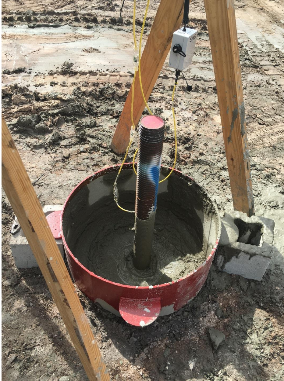
Figure 2.21 Pile T2 with thermal wires and attached TAP unit.
