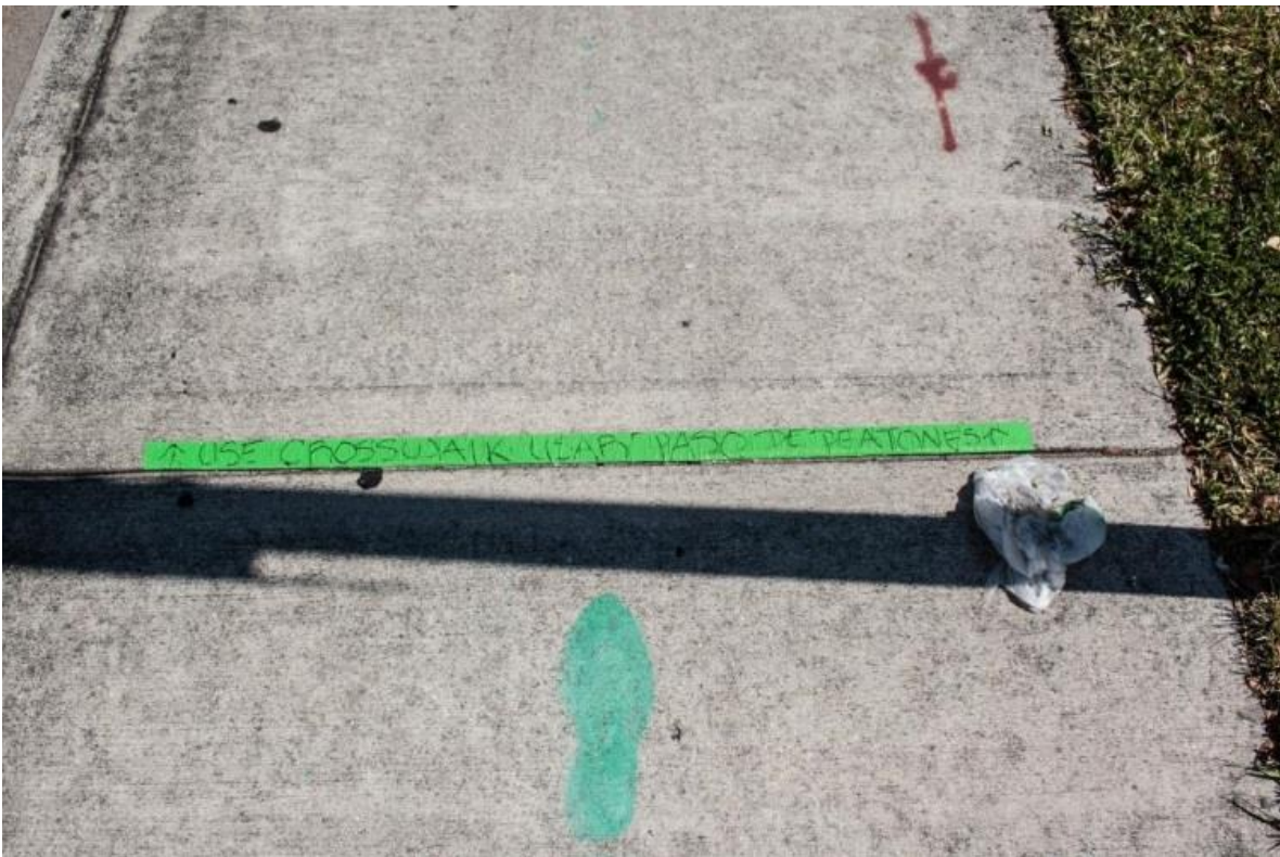
Photo 4-21 Tape on sidewalk directing pedestrians toward crosswalk
