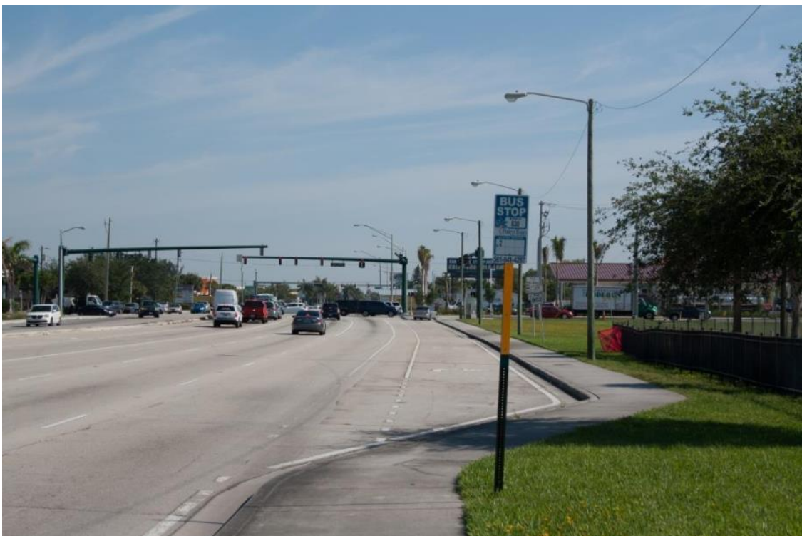
Photo 4-18 Bus Stop 830 is located approximately 530 feet south of Lake Worth Road
