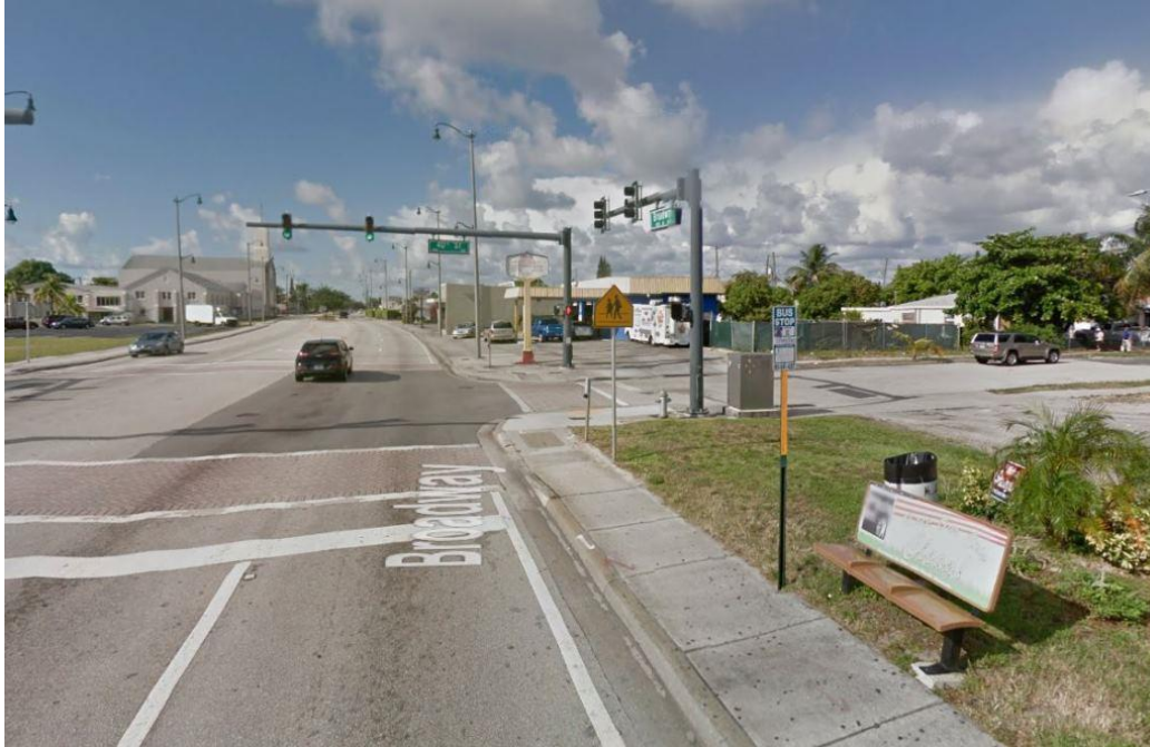
Photo 2-17 Bus Stop 82 (looking south on Broadway)
