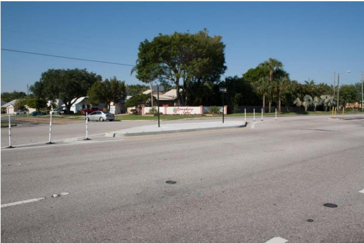
Photo 4-12 There is no easy way to cross Lantana Road at Brentwood Blvd.
