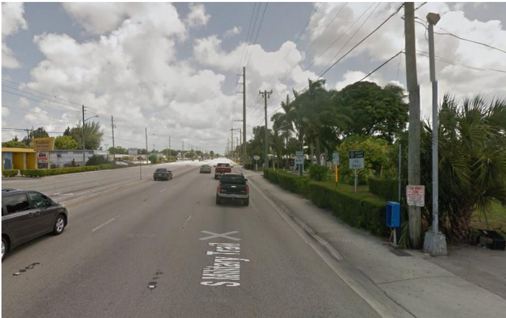
Photo 2-29 Bus Stop 1055 (looking south on S. Military Trail)
