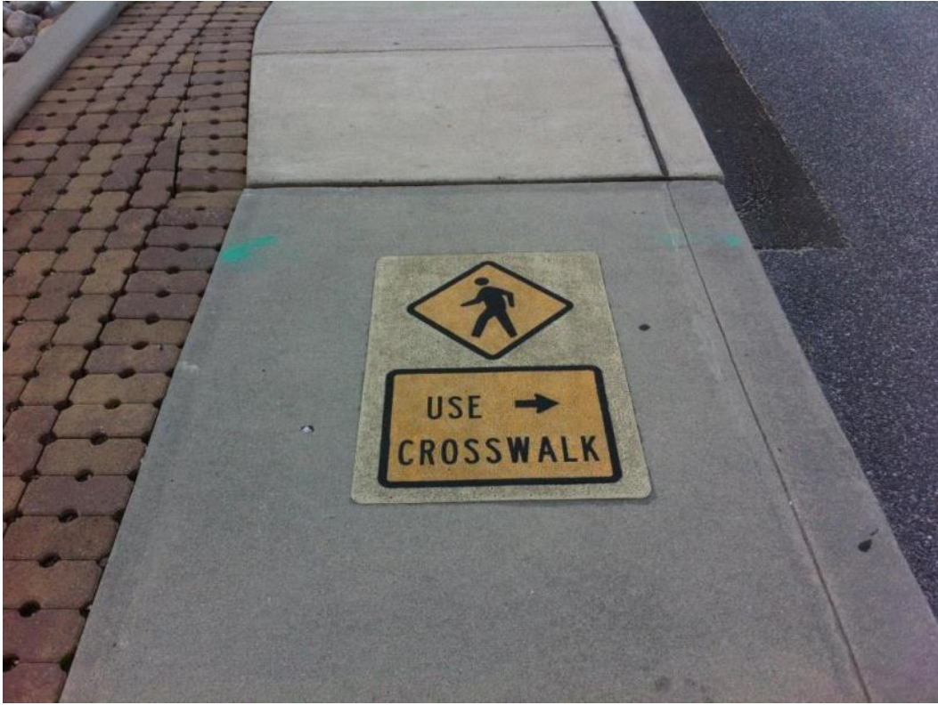
Photo 4-2 "Use Crosswalk" sidewalk stencil
