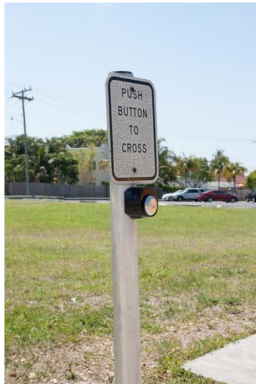
Photo 4-24 Pedestrian push button at Broadway and 40 th Street is out of date
