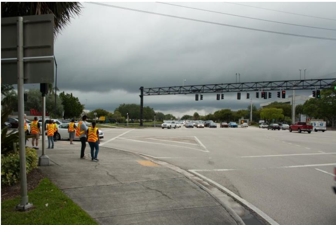
Photo 4-9 Northbound right turn lane has large radius that encourages high speed turns
