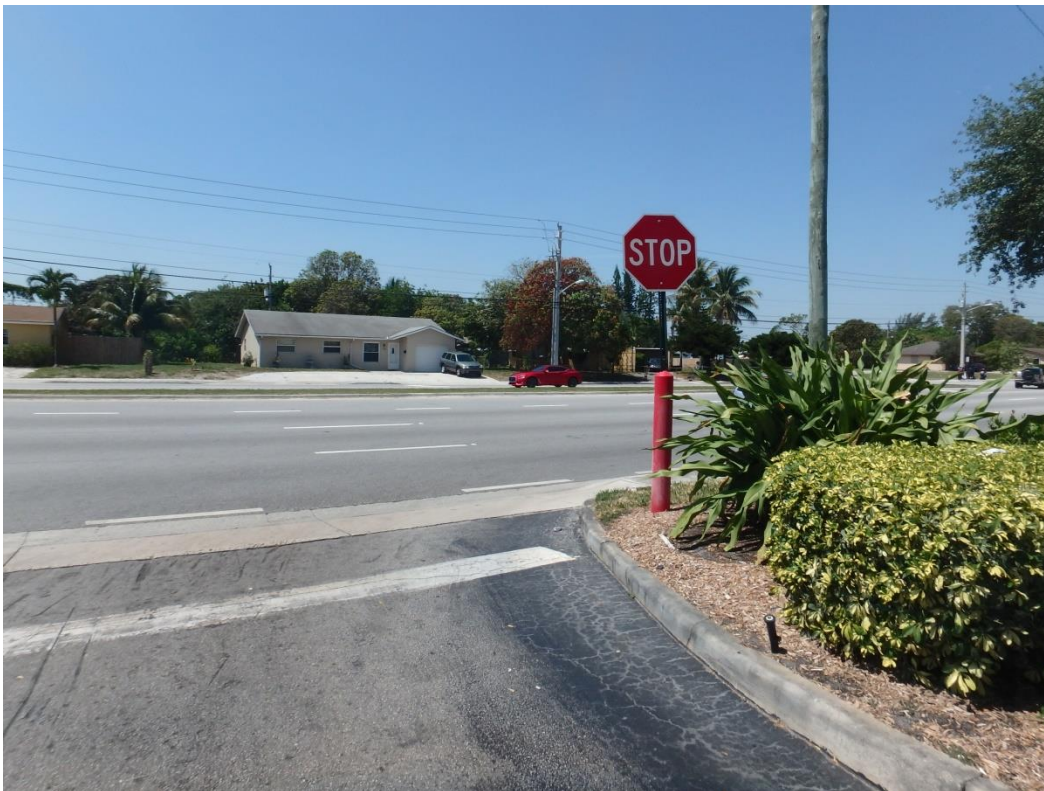
Photo 4-26 No pedestrian warning signs at entrance to Poinciana Plaza
