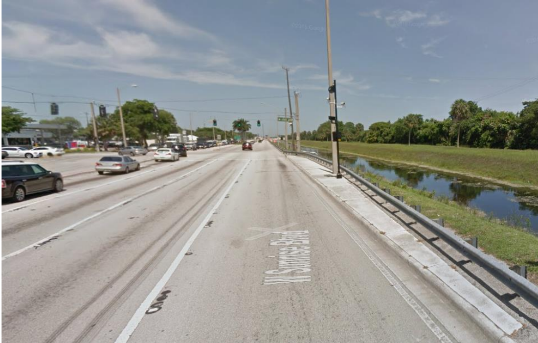
Photo 2-11 Bus Stop 1791 (looking east on W. Sunrise Blvd.)
