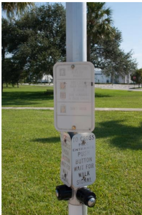
Photo 4-16 Pedestrian signal push button signs near the entrance to Palm Beach State College are faded
