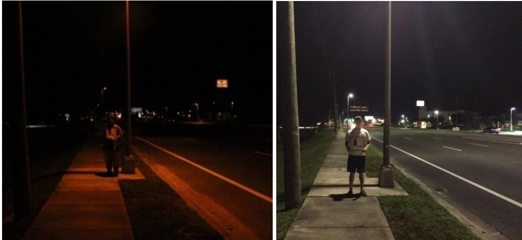
(a) Before: High pressure sodium (HPS) (b) After: Light-emitting diode (LED)
