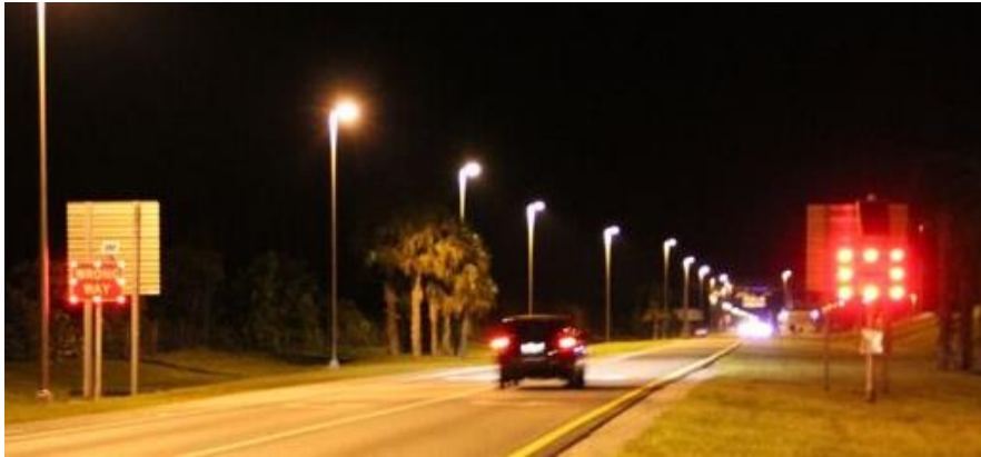
Figure 28: Detection-Triggered LED Lights around “WRONG WAY” Signs
