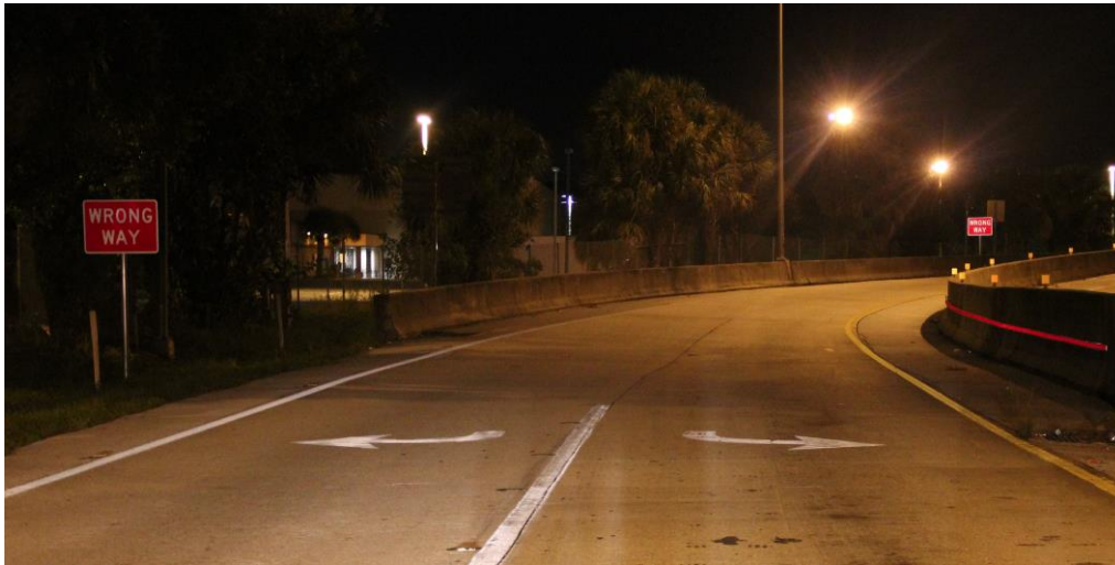
Figure 32: Delineators along Off-ramps
