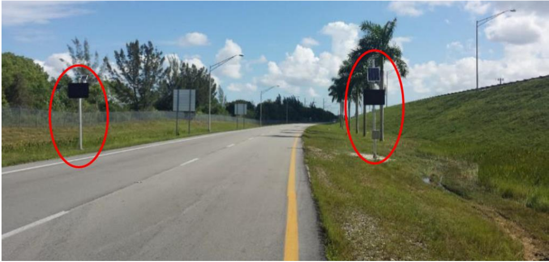
(a) Off-ramp with LED-illuminated “WRONG WAY” sign location
