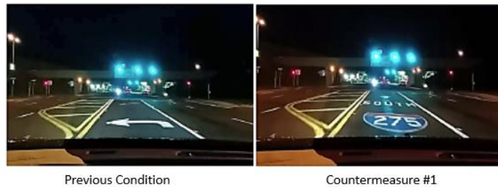
Figure 74: Newly-developed S&PM Standards – WWD Countermeasure #1
