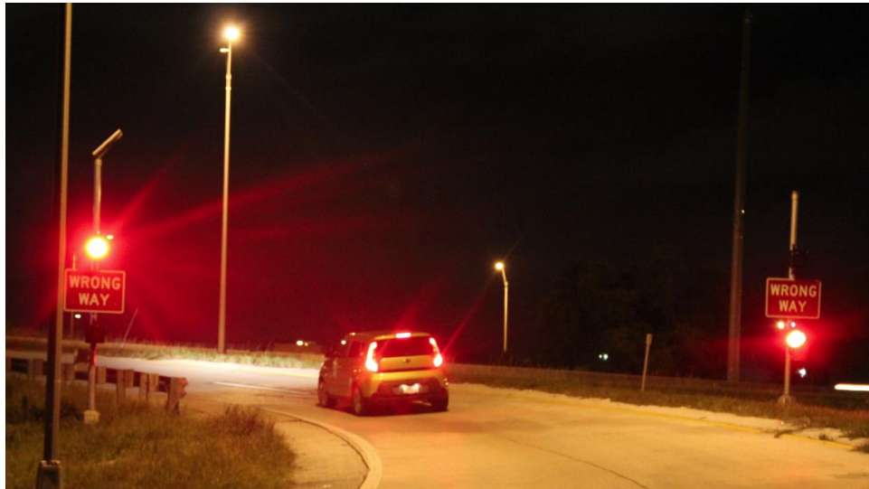
Figure 34: Wigwag Flashing Beacons
