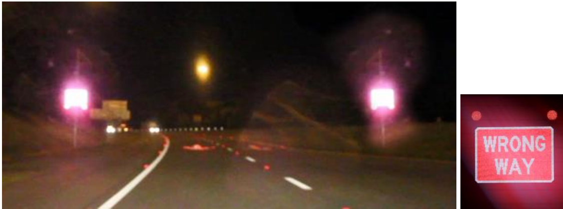
Figure 30: Detection-triggered Blank-Out Signs That Flash “WRONG WAY”
