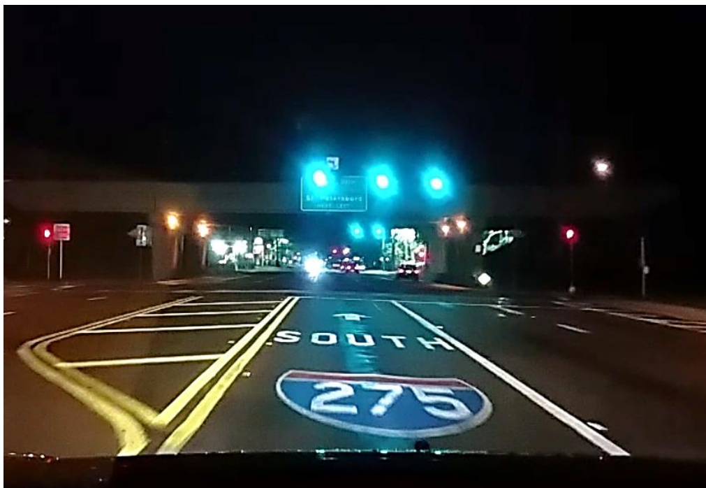
Figure 22: Newly-developed S&PM on Arterials to Mitigate WWD
