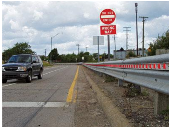
Figure 15: Delineators along Off-ramps
