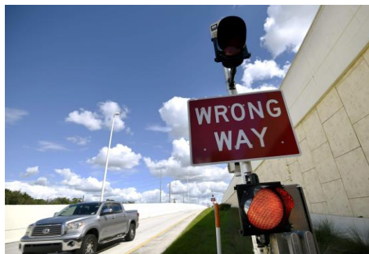
Figure 16: Wigwag Flashing Beacons
