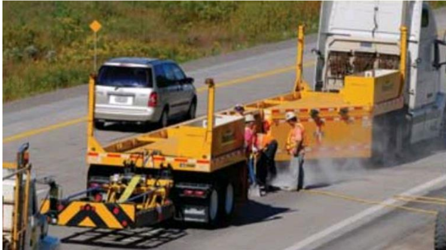
Figure 4-5 Using MBT-1 mobile work zone barrier in the field (Graham et al., 2011)
