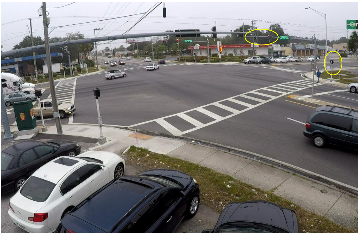
Figure 4-27 Field data collection after LPI implementation at E Fletcher Ave @ N Nebraska Ave, Tampa, FL (GoPro view).
