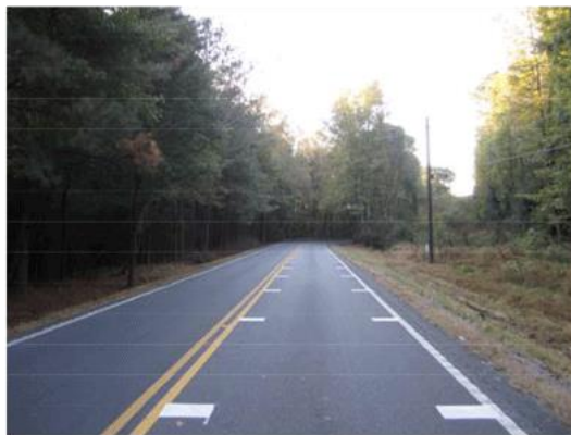
Figure 44. Example of Speed Reduction Markings
