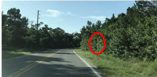
Obstruction at Site 8 (WB, 28°50'02.1"N 82°40'19.4"W)
