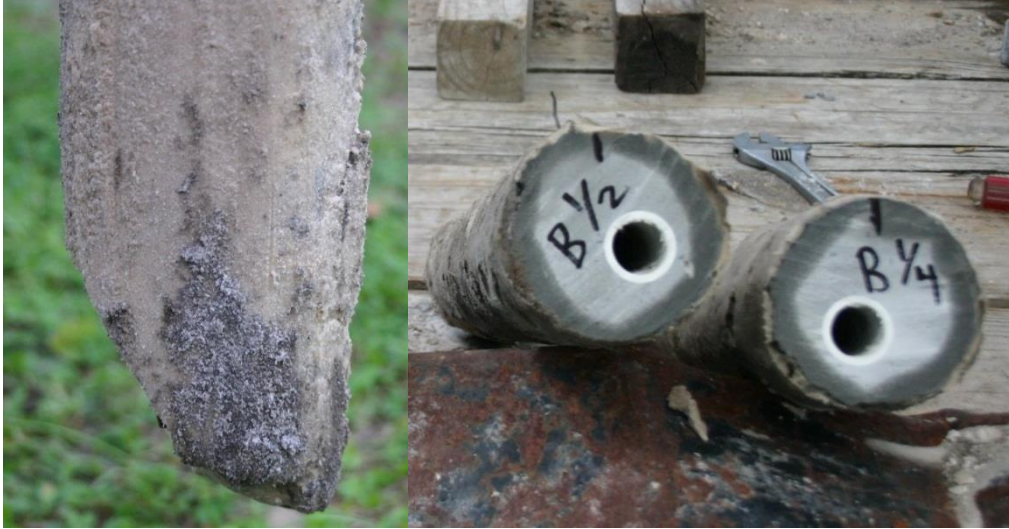
Figure 3.81 saturated soil on shaft perimeter (left), ring of moisture in cross section of shaft (right).
