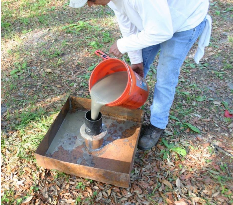
Figure 3.42 Slurry introduction into the borehole.
