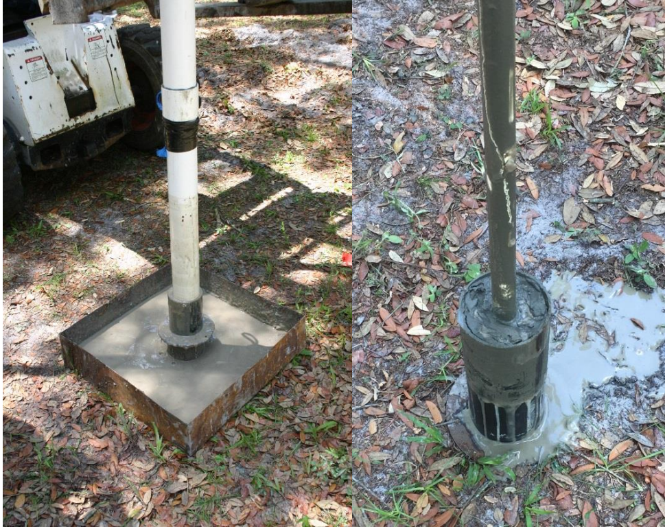
Figure 3.48 Mortar expelling slurry (left), fully concrete shaft (right).
