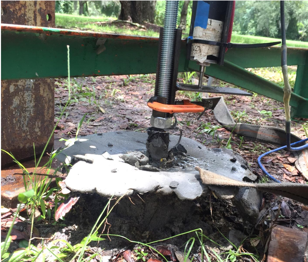
Figure 3.52 Static load test of shaft.
