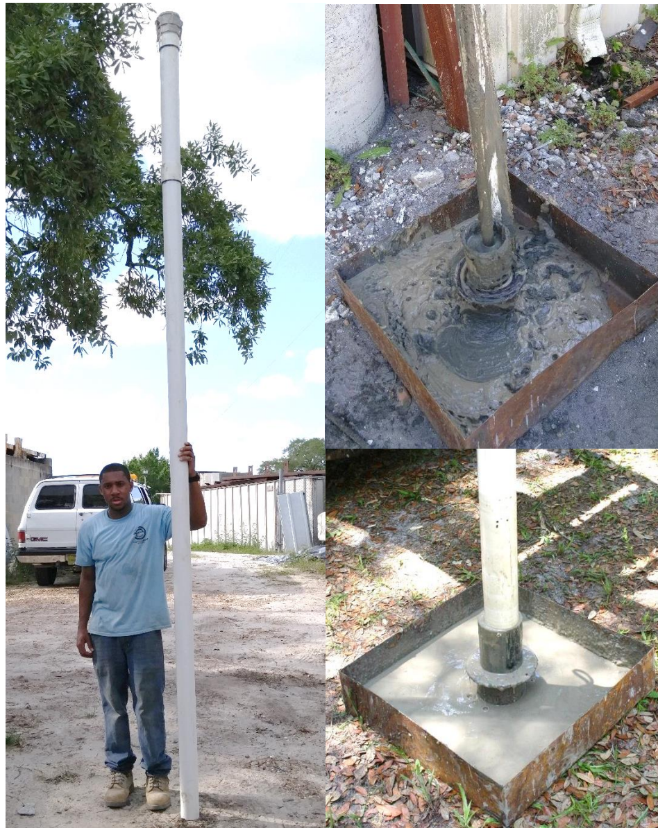
Figure 3.14 Twelve foot long, 3in diameter tremie (left), poor slurry displacement with 2in tremie (top right), improved slurry displacement with 3in tremie (bottom right).
