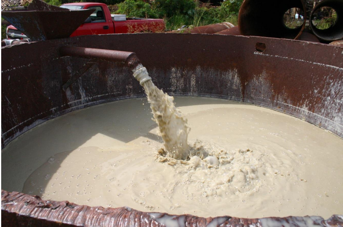
Figure 4.9 Bentonite slurry ready for use immediately after mixing.
