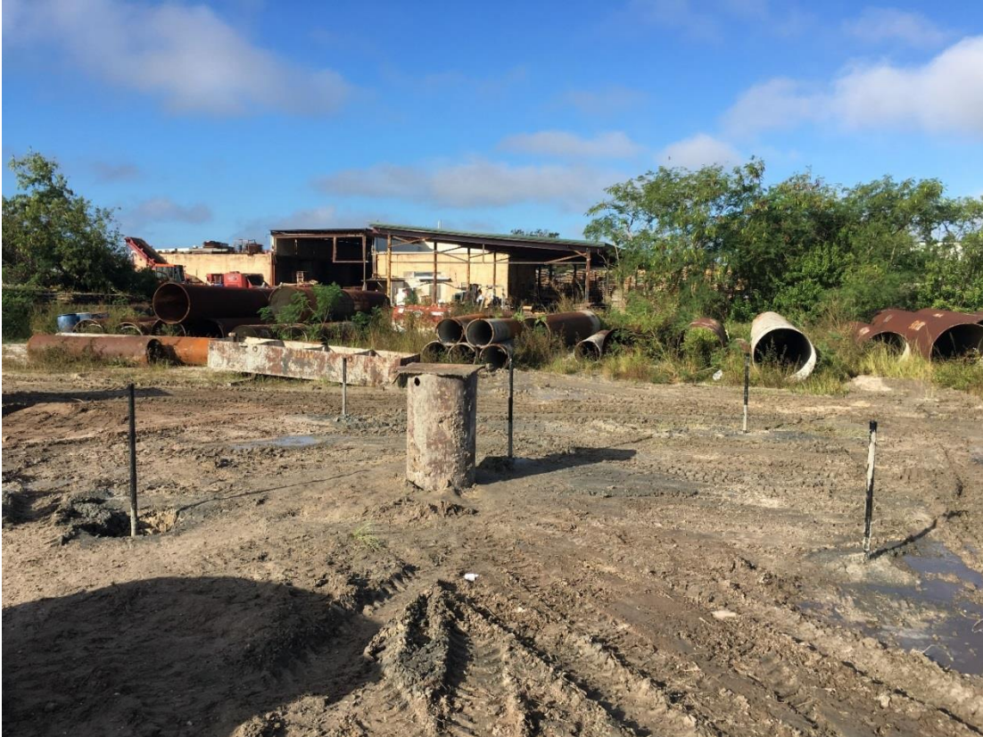
Figure 4.23 All shafts completed and site back-bladed clean (short casing not embedded).
