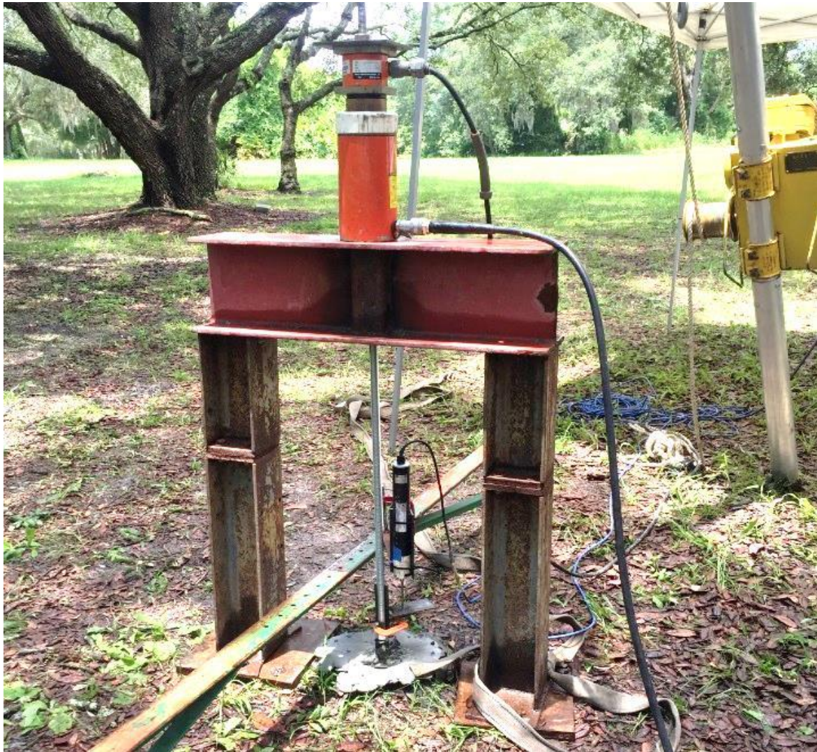
Figure 3.51 Pullout static load testing apparatus.
