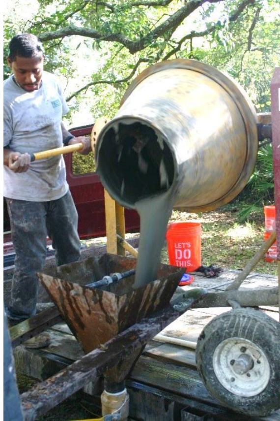
Figure 3.45 Mortar mix being transferred to the hopper.
