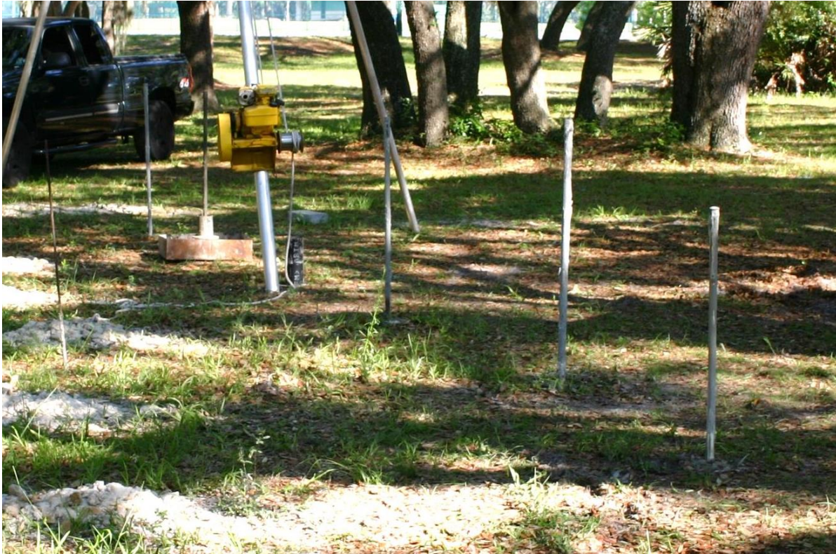
Figure 3.50 Concreted bentonite shafts.
