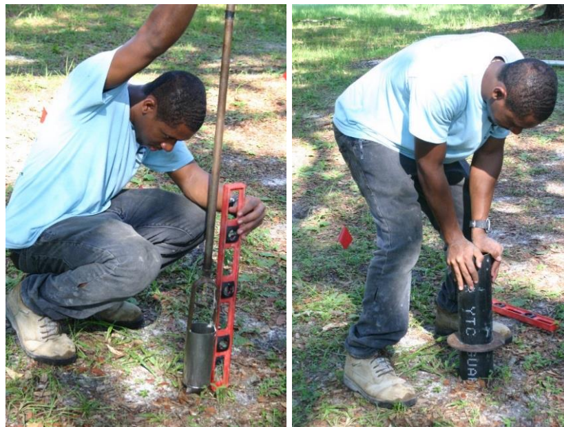
Figure 3.41 Levelling the hand auger (left), casing installation (right).
