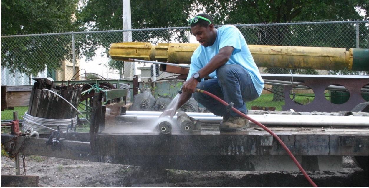
Figure 3.58 Filter cake removal of shaft quarters.
