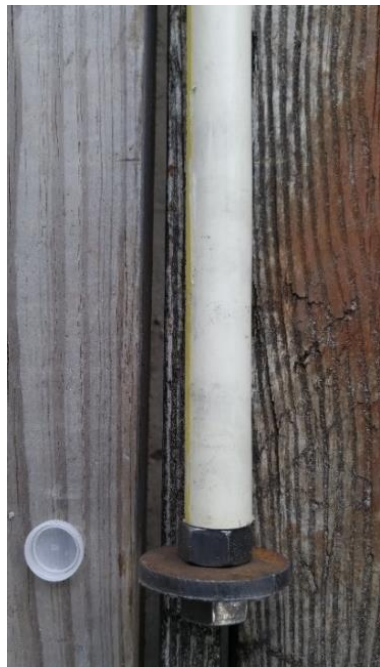
Figure 3.12 Bottom plate secured with \frac{3}{4} in nuts.
