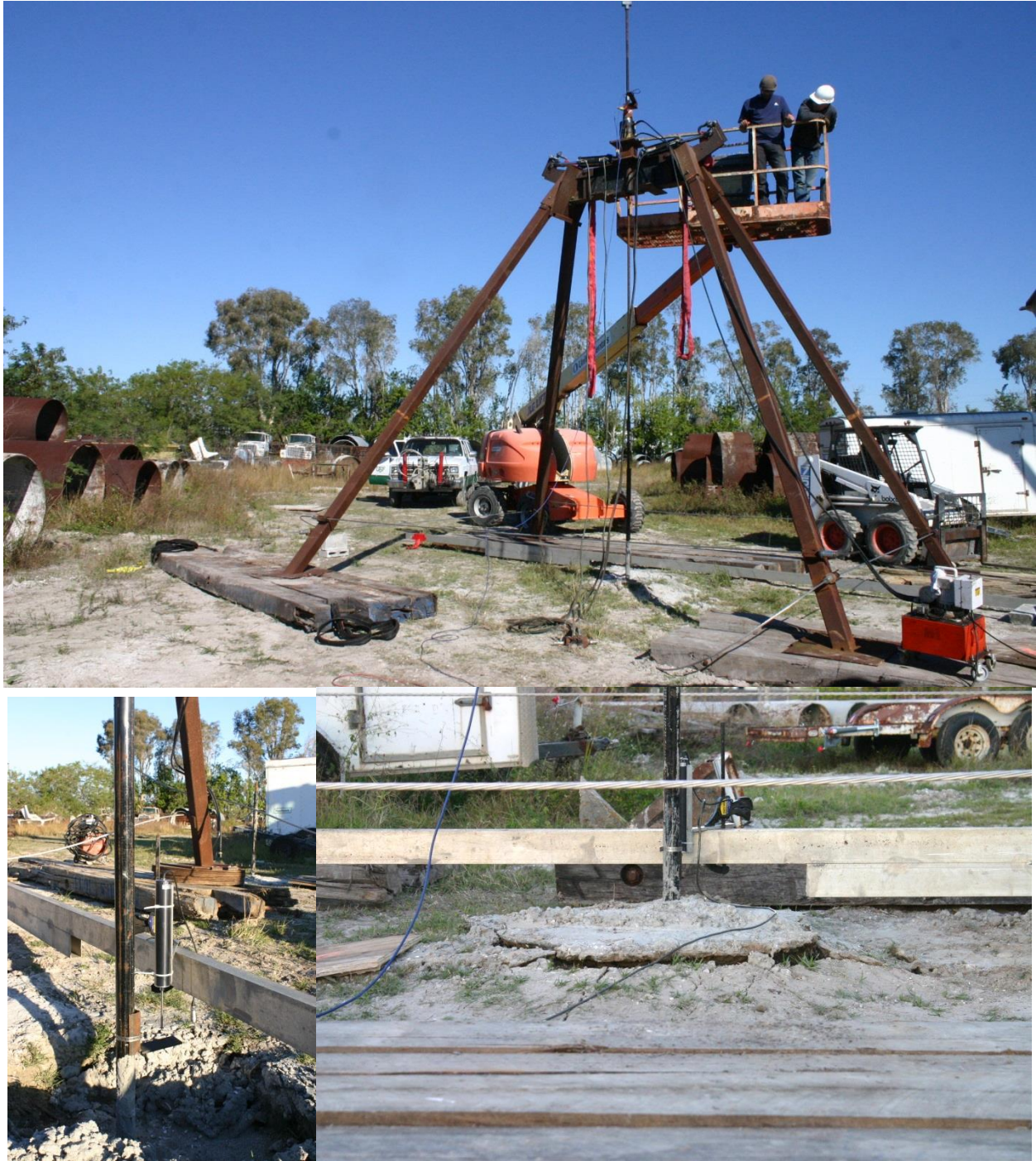
Figure 4.27 Load testing in progress.
