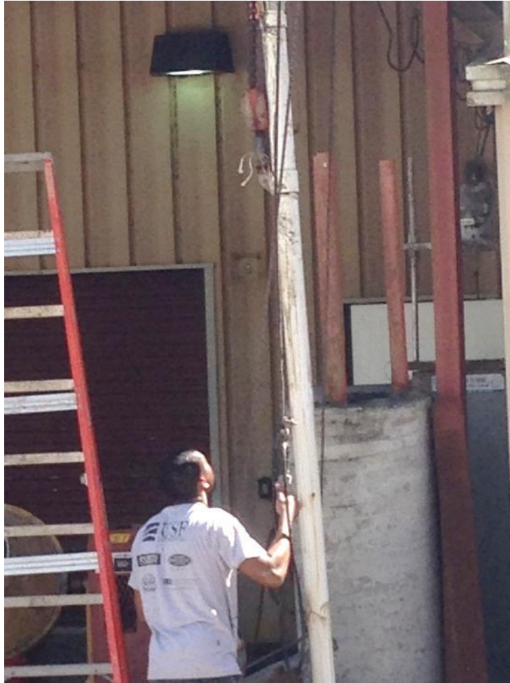
Figure 3.15 Tremie extraction with electric hoist during mock test.
