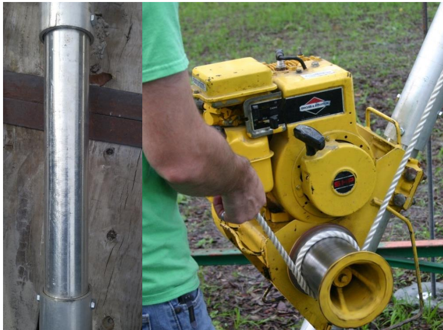
Figure 3.17 Modified tripod leg (left) mounted cathead in operation (right).
