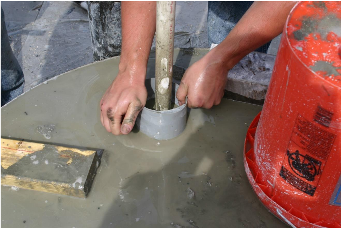
Figure 3.16 Debonding plastic sleeves on top 8in of the sockets.
