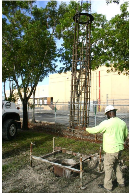
Figure 4.12 Cage installation: control shaft (left) and temporary cased shaft (right).
