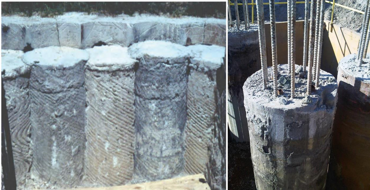
Figure 1.1 Surface texture from rotating casing during extraction (left, FHWA 2010); smooth surface from vibratory extraction (right).
