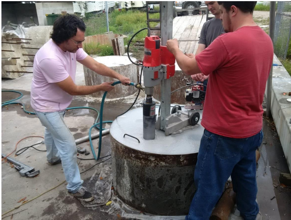
Figure 3.8 Top of simulated limestone beds flooded with water and being pre-cored.
