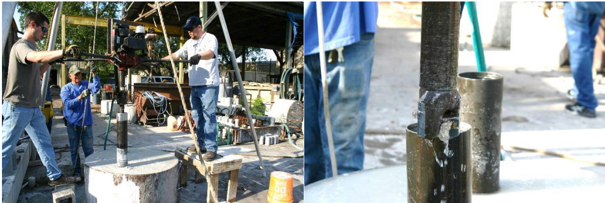
Figure 3.11 Rotatory casing installation (left) and drill bit (right).
