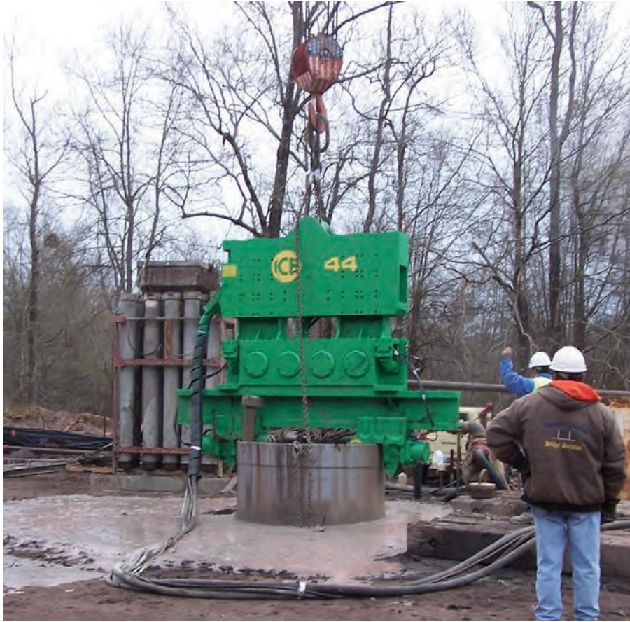
Figure 2.14 Casing extraction using vibratory hammer (FHWA, 2010).
