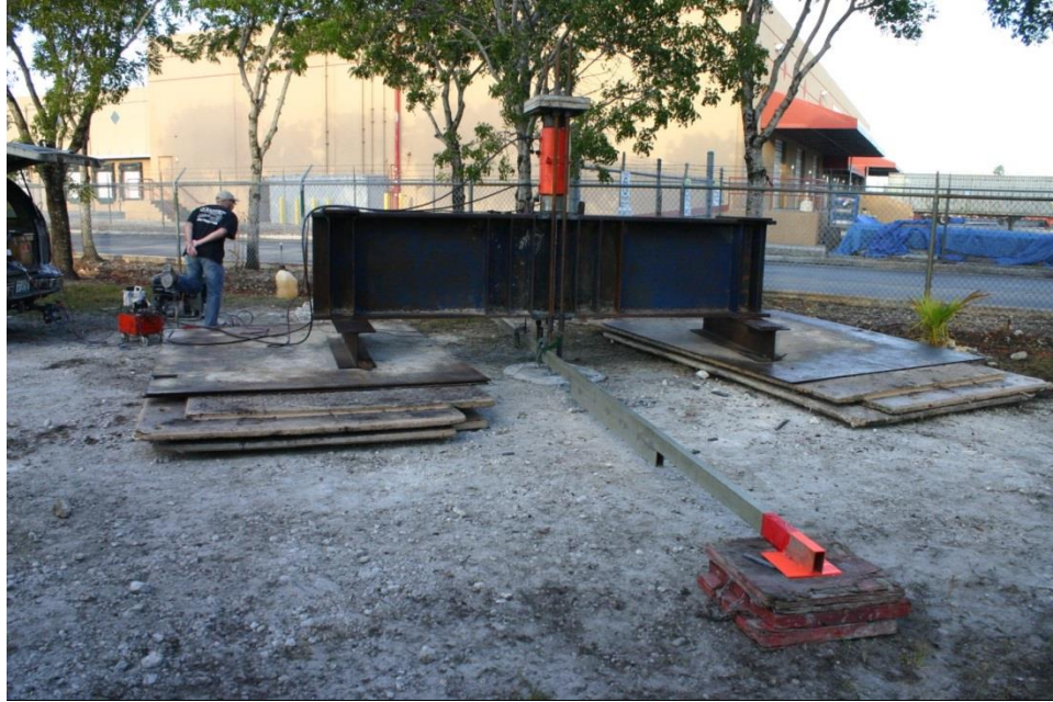
Figure 4.18 Completed loading system with reference beam.
