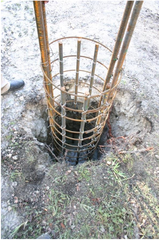
Figure 4.12 Cage installation: control shaft (left) and temporary cased shaft (right).
