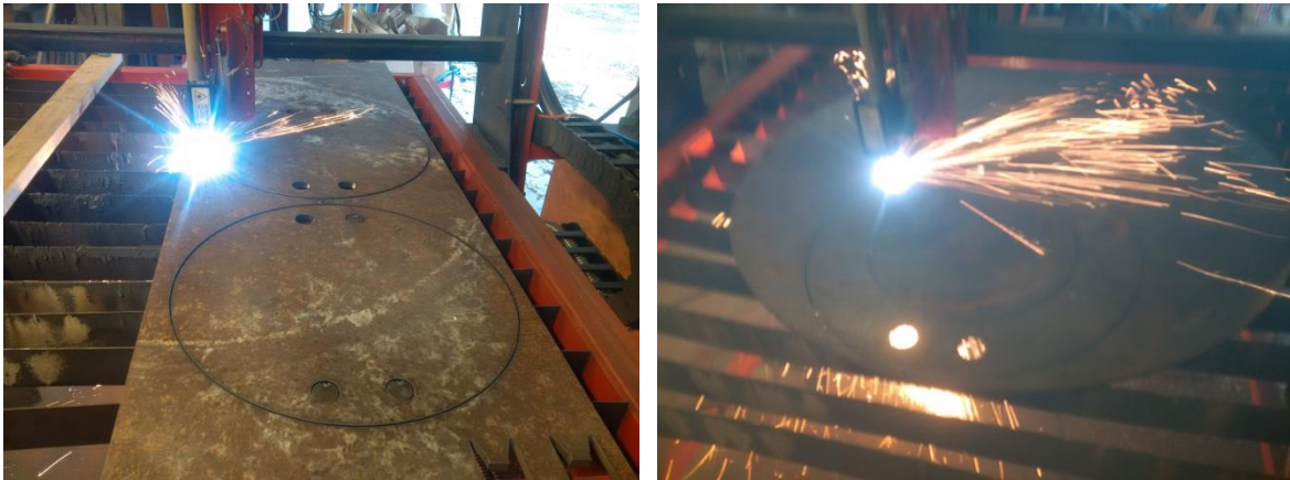
Figure 4.6 Base plates (left) and upper spacer plates (right) being cut out.
