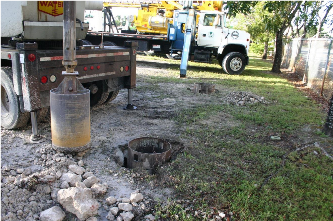
Figure 4.10 Both shafts after excavation and casing advancement.
