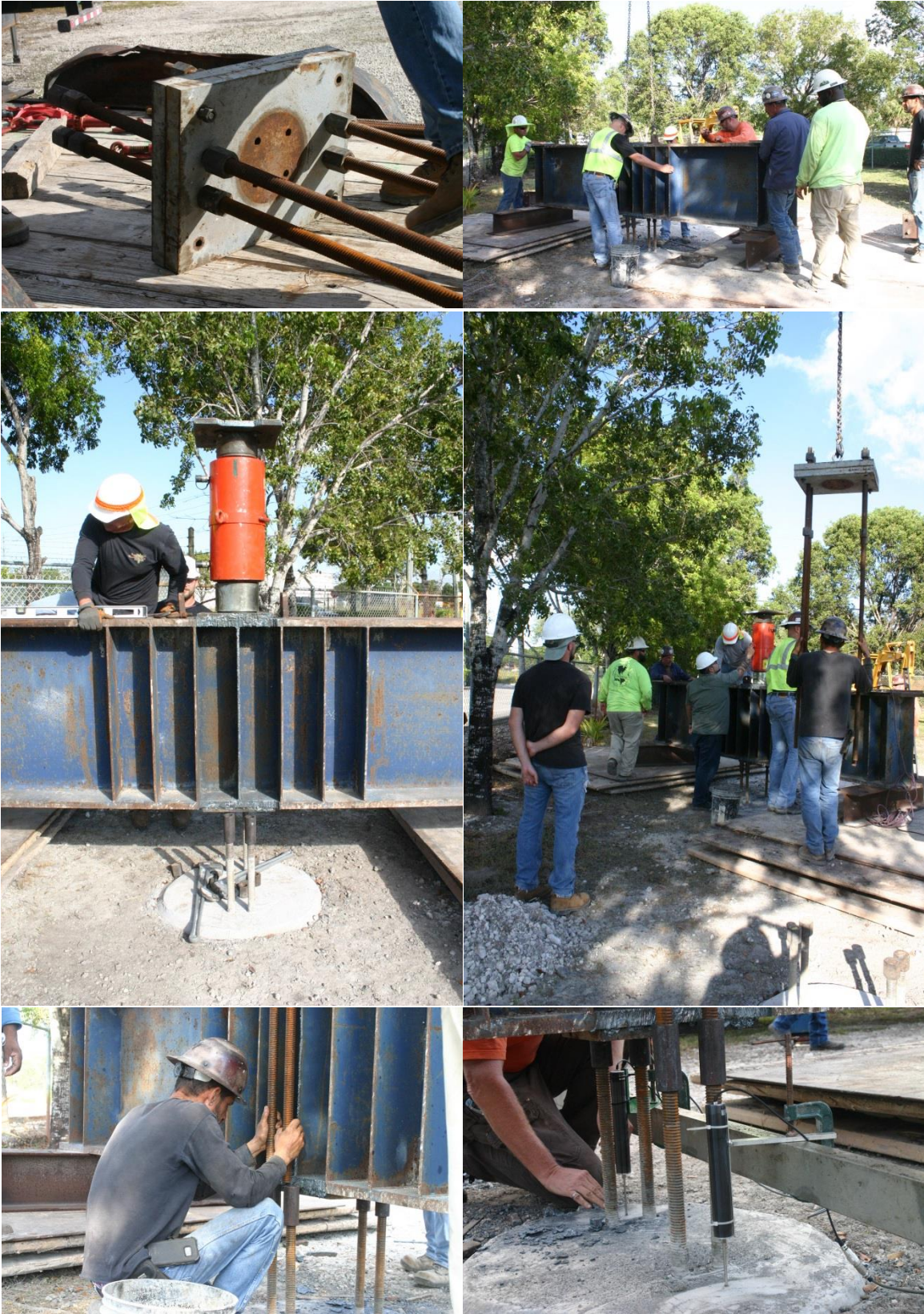
Figure 4.17 Load test setup.
