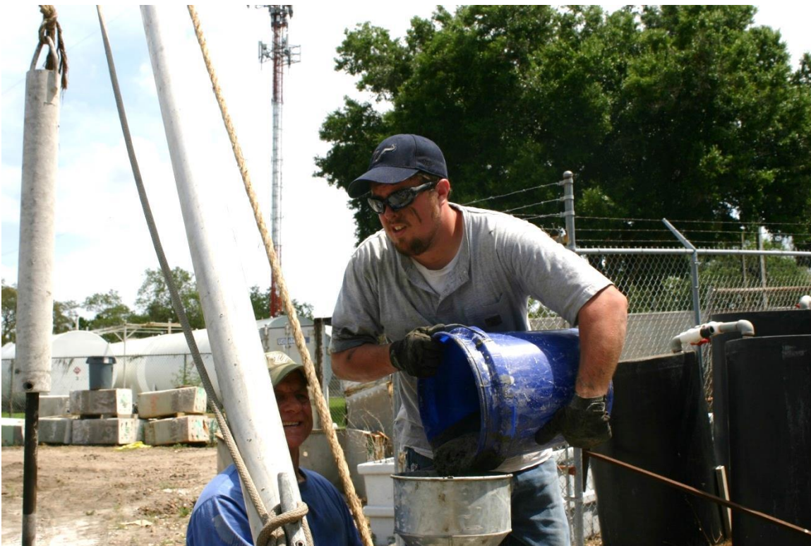
Figure 3.14 Filling tremie and hopper while casting rock sockets.
