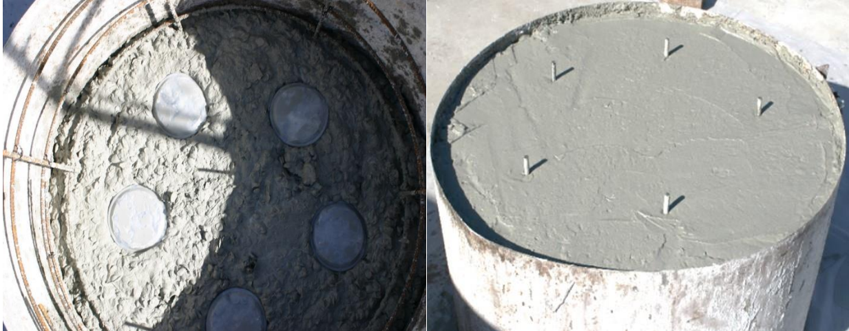
Figure 3.3 Debonding plastic disks (left) and centering rods (right).
