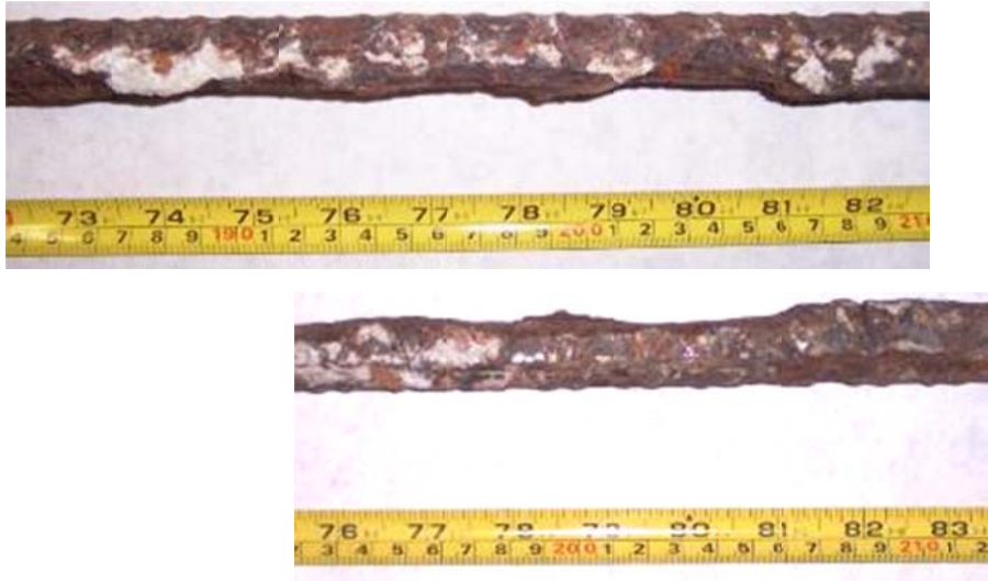
Figure 15. Corrosion-related cross-section loss in Bar #5.
