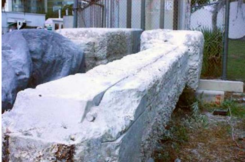
Figure 8. Vertical and horizontal saw cuts in the submerged portion of Pile #2.
