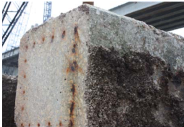
Figure 22. Submerged (i.e., bottom) end of extracted pile, oblique view. Note that marine growth has been scraped from the surfaces near the corner to facilitate saw cuts.
