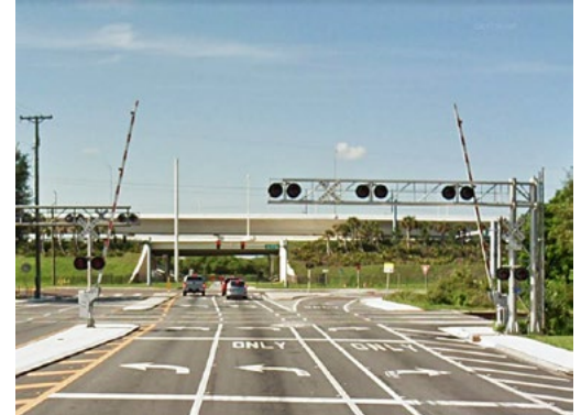
Some drivers approaching this intersection have responded to the turn lane markings with an improper turn onto the railroad tracks.
