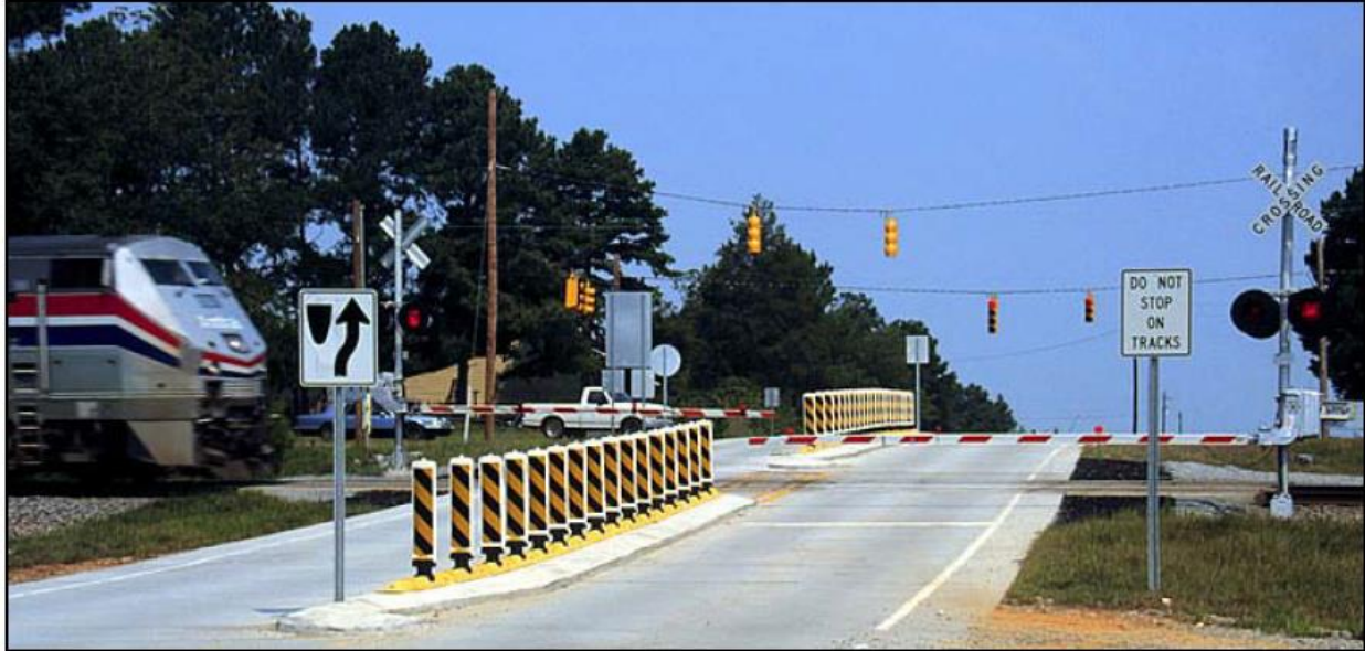
Figure 1-9 Example of Qwick Kurb at railroad crossing ( photo courtesy of NCDOT ).
