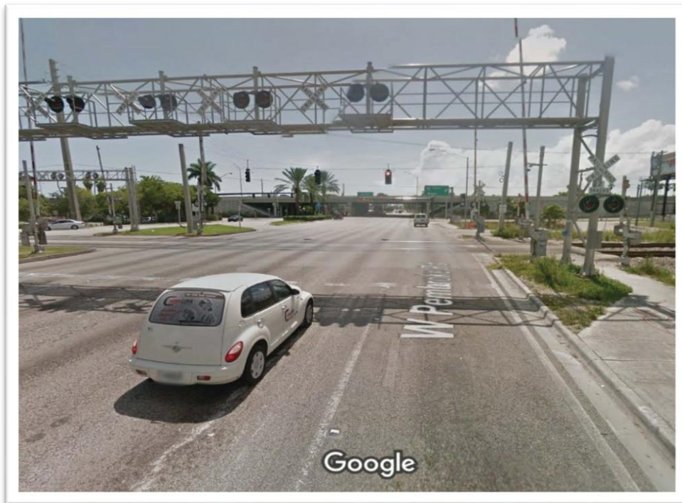
Figure 4-14 W Pembroke Rd @ I-95, Street View.
