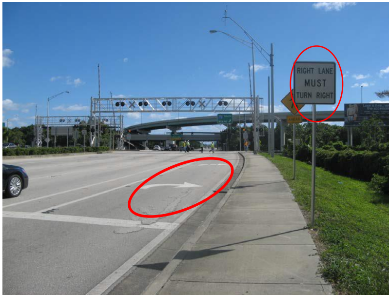
Figure 1-2 Example of potentially misleading right-turn sign and pavement markings.
