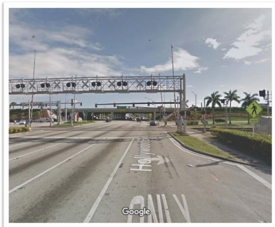
Figure 4-6 Hollywood Blvd @ I-95, Street View.
