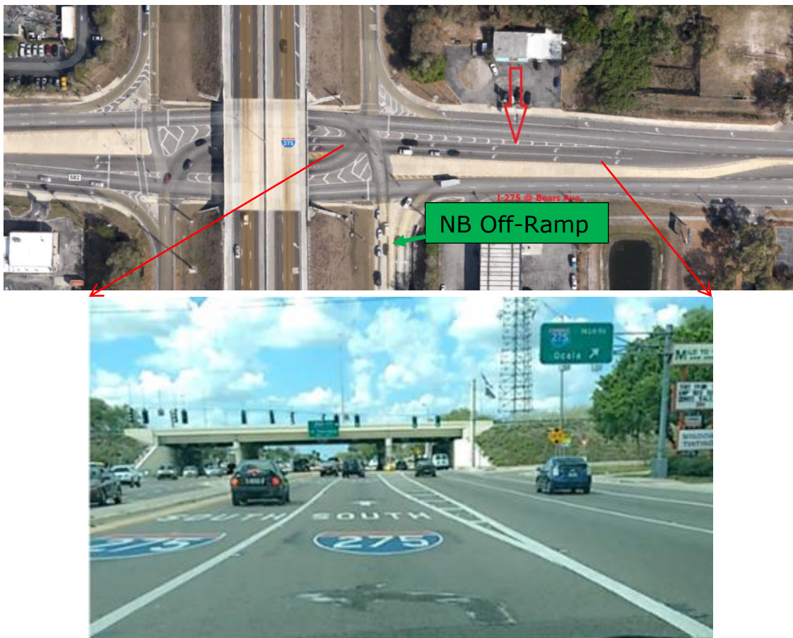
Figure 1-4 Pavement markings with guidance information at I-275 NB off-ramp at Bearss Ave, Tampa, Florida.
