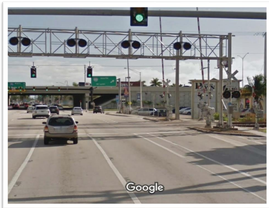
Figure 4-10 W Hallandale Beach Blvd @ I-95, Street View.
