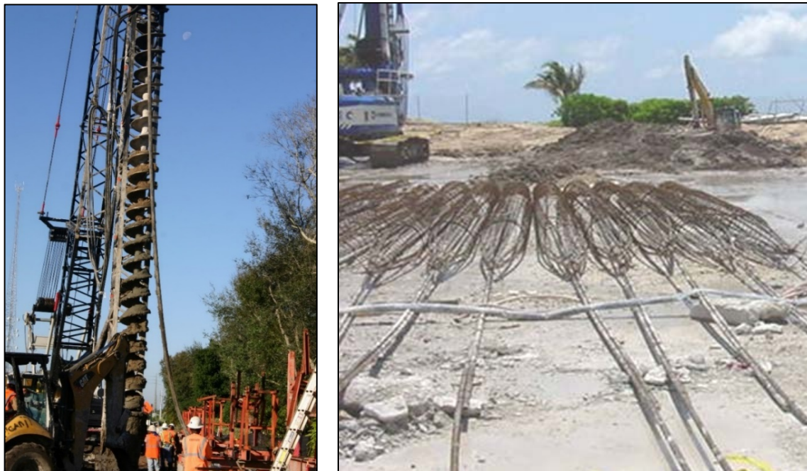
Figure 2.1. ACIP drill rig (left) and pile reinforcement (right)
