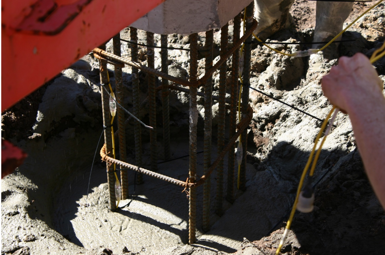
Figure 5.35. Cage instrumented with two wires being placed into grout
