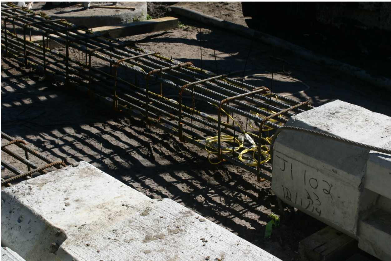
Figure 5.34. ACIP reinforcing cage instrumented with four thermal wires
