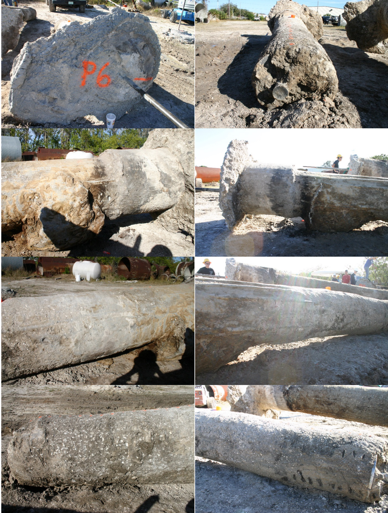
Figure B.10. Shaft P-6 (from top to bottom): shaft top (left) and toe (right); side views of shaft top section; side views of shaft middle section; side views of bottom section
