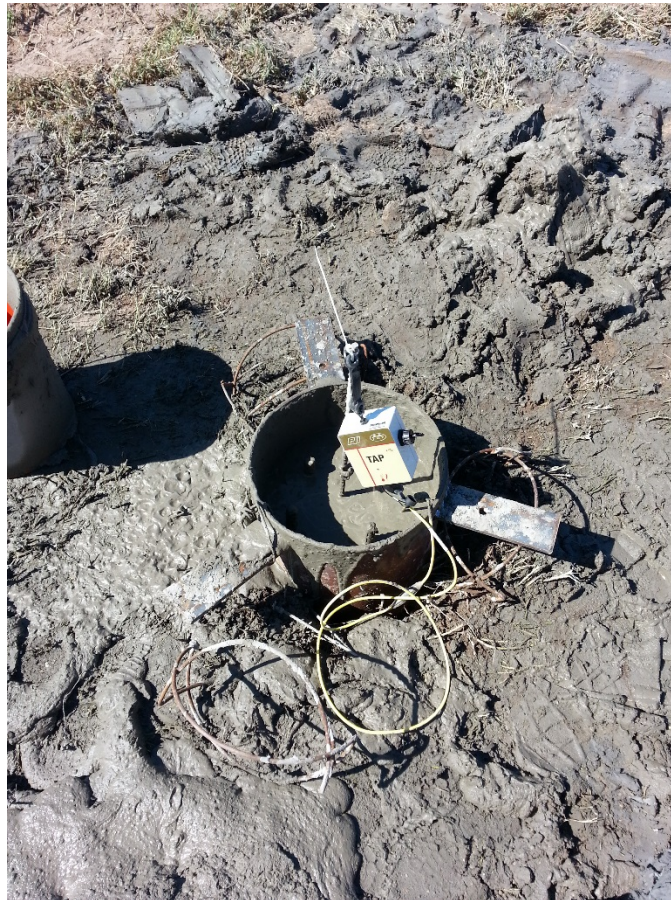
Figure 5.21. 14in ACIP pile instrumented with single center thermal wire
