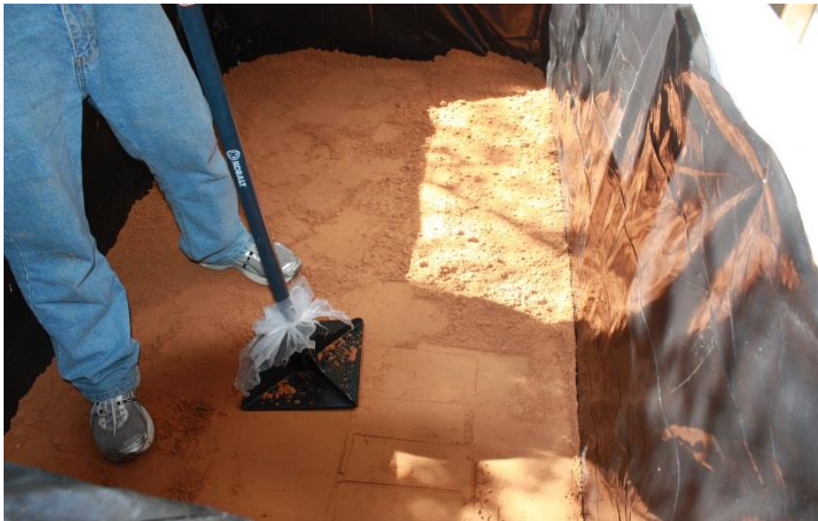
Figure 21. Compacting backfill in soil box.
