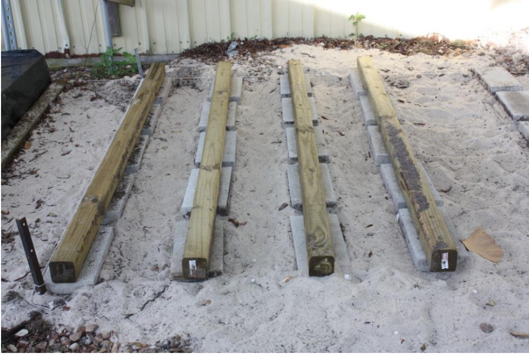
Figure 16. Foundation of the soil boxes.
