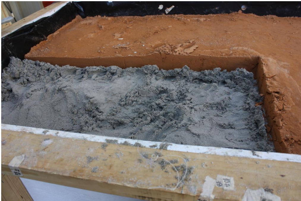
Figure 27. Complete removal of the dam before CLSM top-up.
