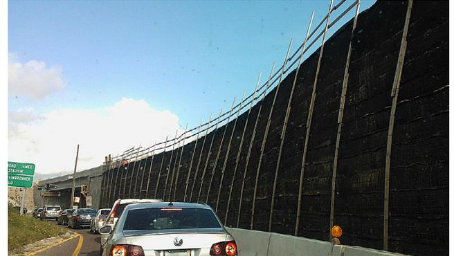
*The black wall (right) is an earthwork, retained by geotextile, which supports a section of I-295 under construction.*
