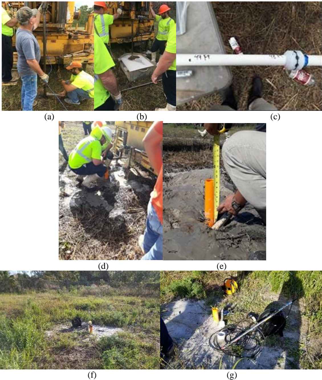
Figure 3-5. (a) Installation of piezometers in the ground using sacrificial tips, (b) drilling and grouting for installation of magnetic extensometers, (c) magnetic extensometer and datum magnet sensor, and (d-g) inclinometer casing installation
