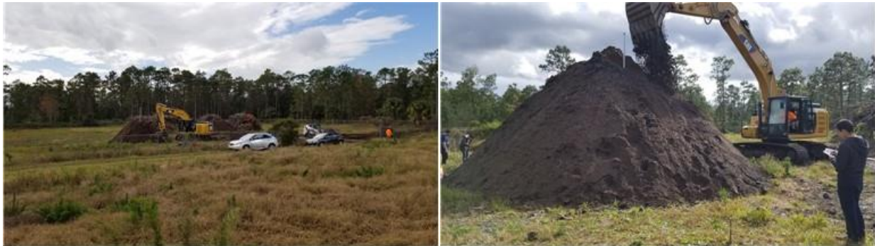
Figure 3-17. Loading sequence after third riser pipe was coupled
