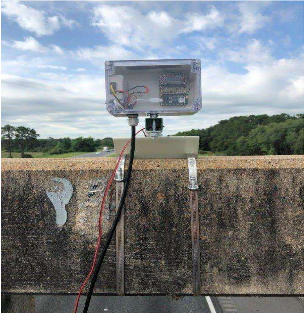
Figure 98: Site 2: Gateway Unit
