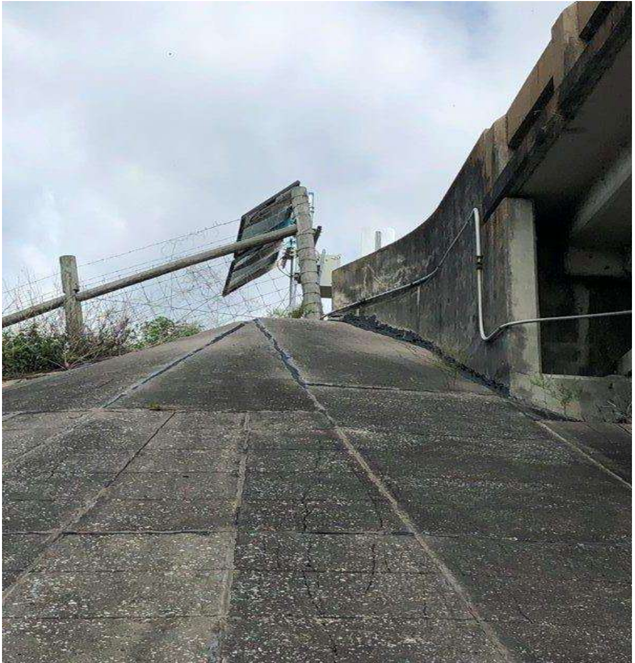
Figure 86: Solar Unit: Site 2
