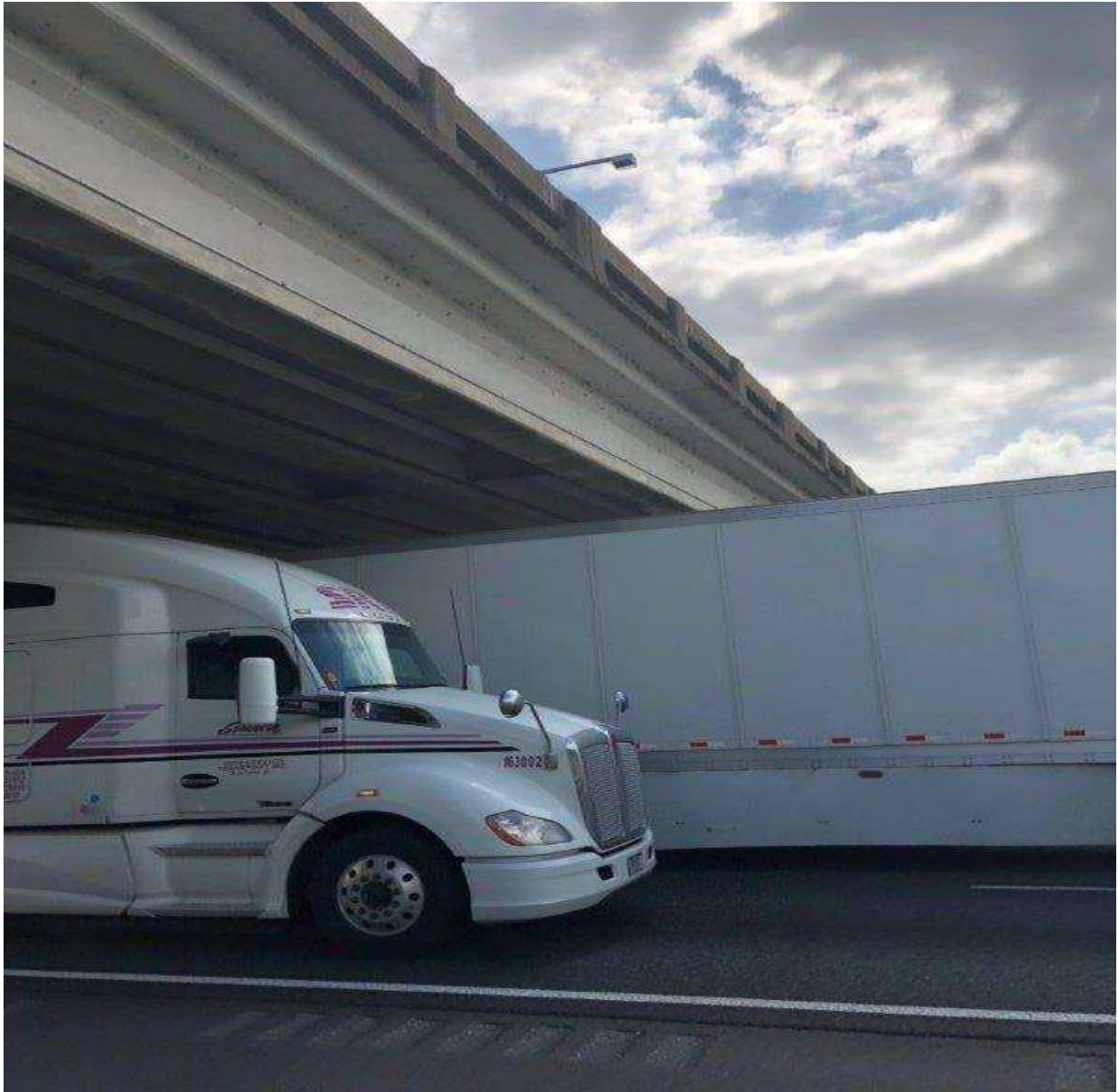
Figure 89: Capture Unit above Traffic
