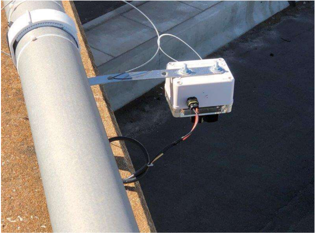
Figure 70: Sensor Looking Down on Traffic
