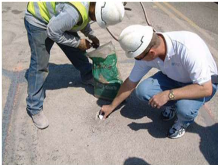
Figure 2: Wireless Magnometer and the Installation Process
