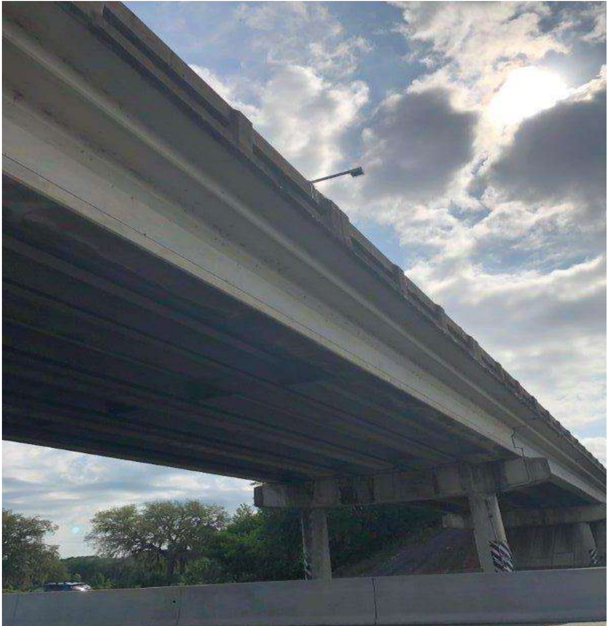
Figure 88: Capture Unit above Traffic
