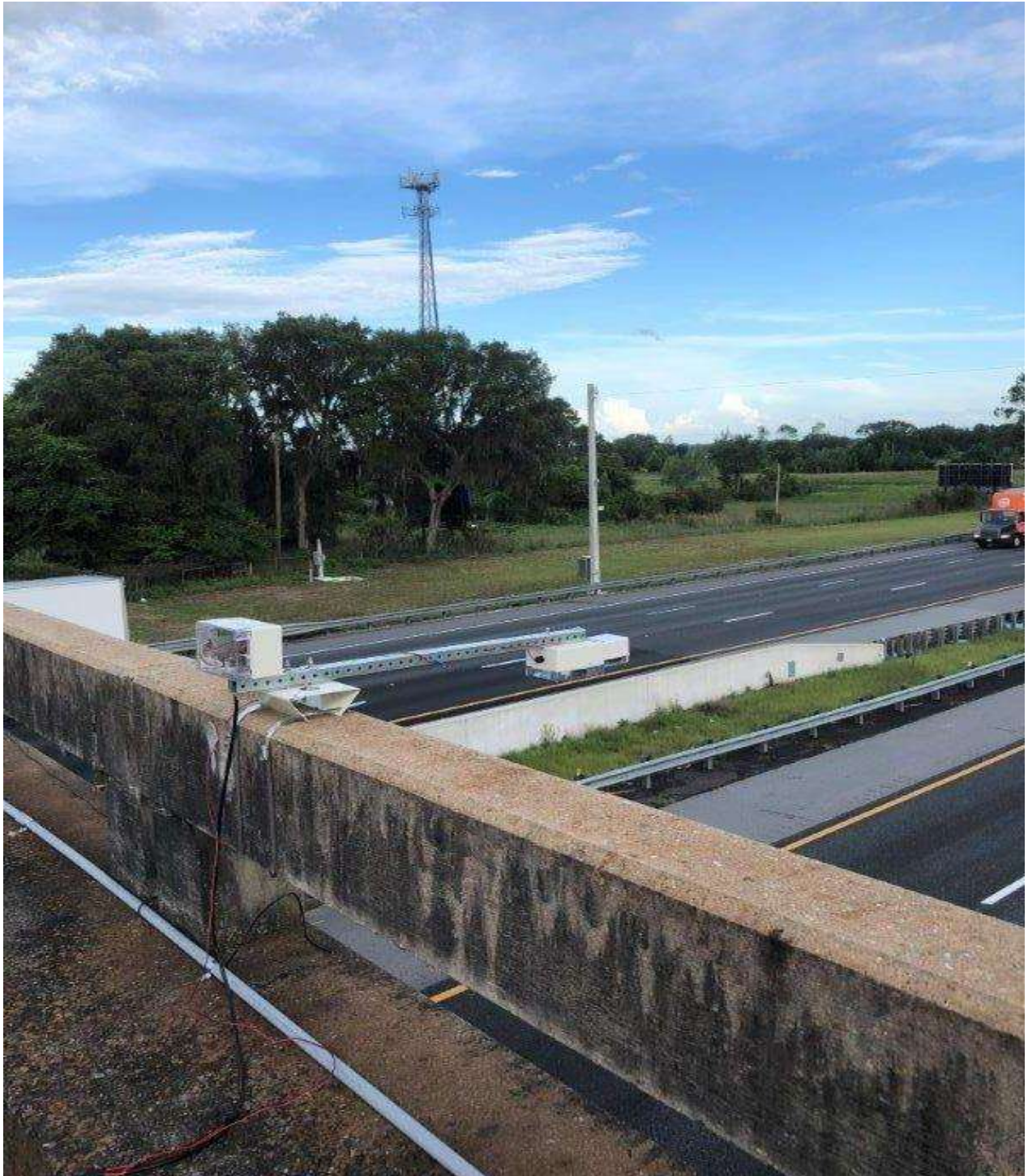
Figure 100: Site 2: Gateway Unit
